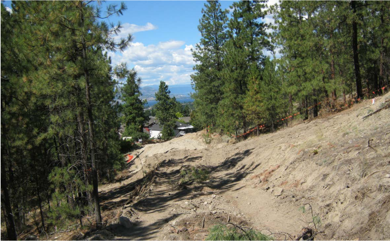
Figure 3: Image of emergency egress road under construction
