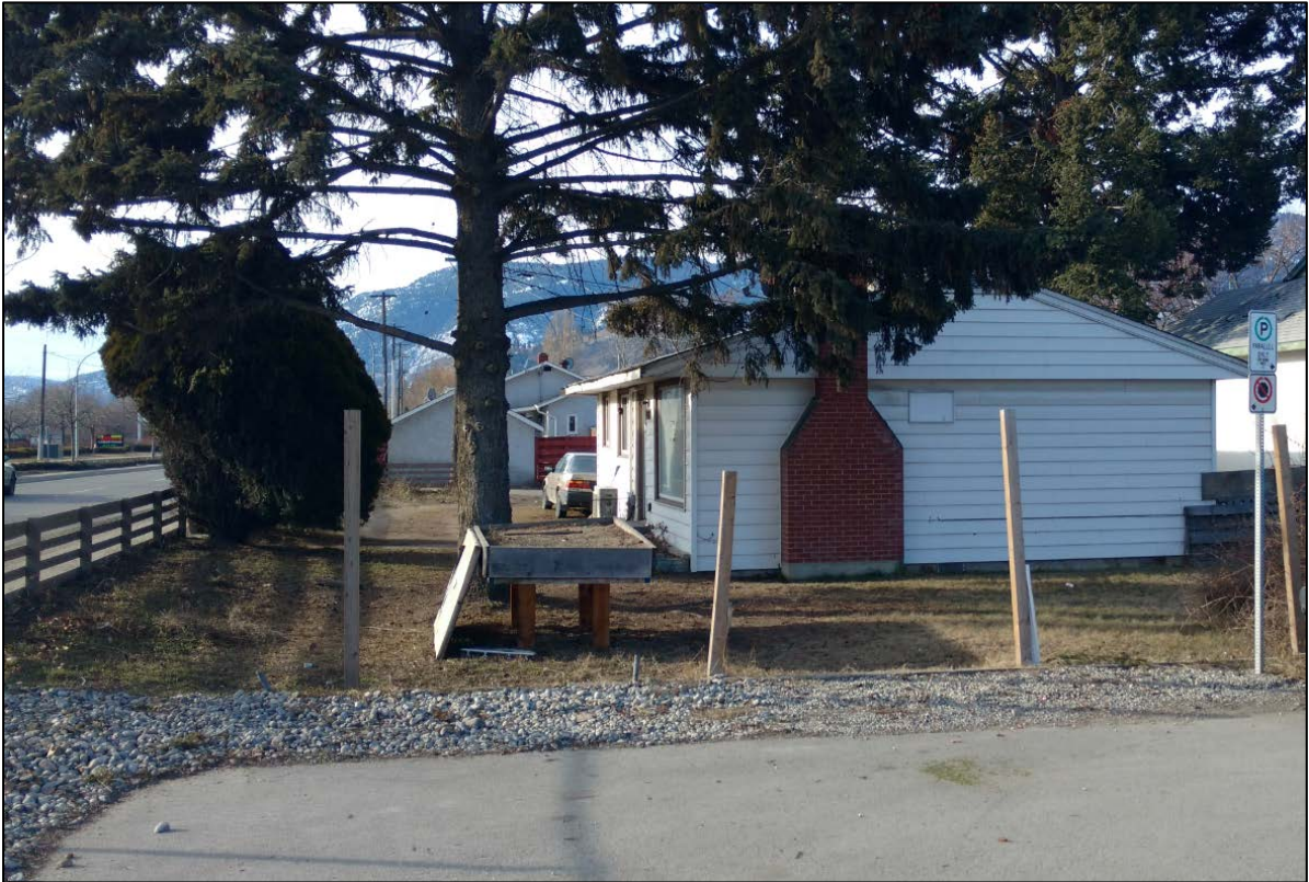
Figure 4: North View (from Revelstoke Avenue)
