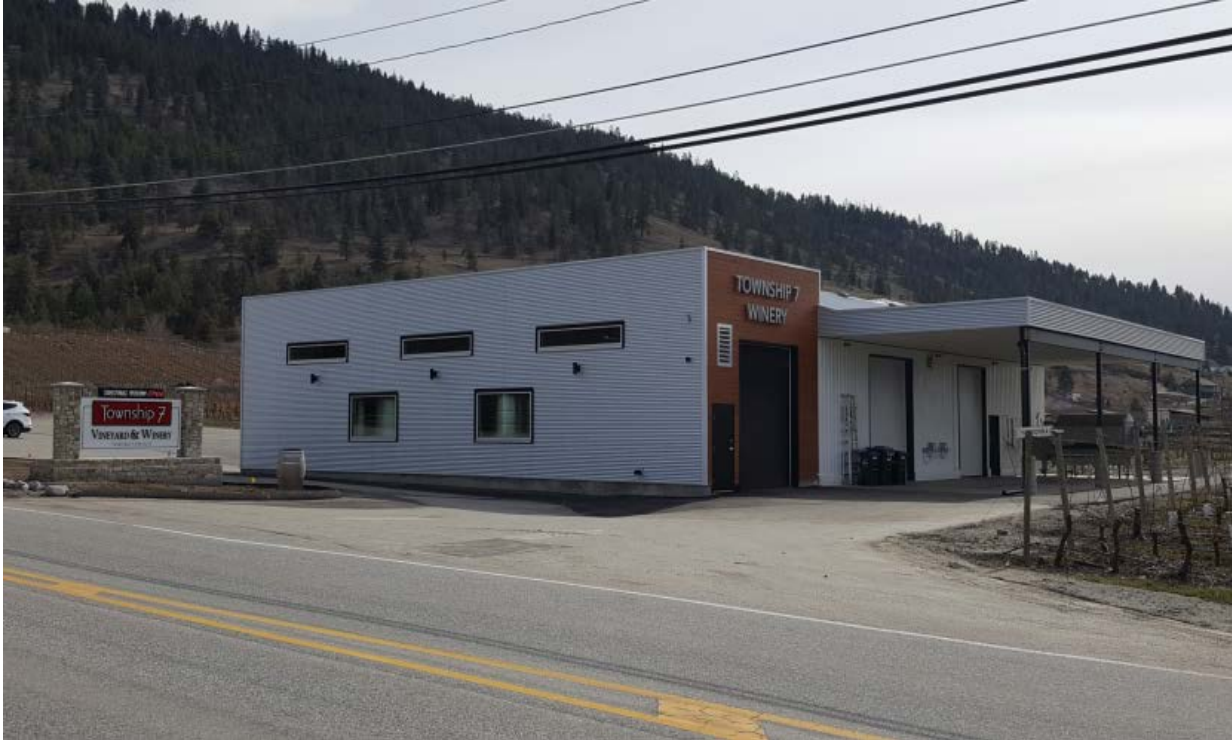
Existing Expanded Building – McMillian Ave
