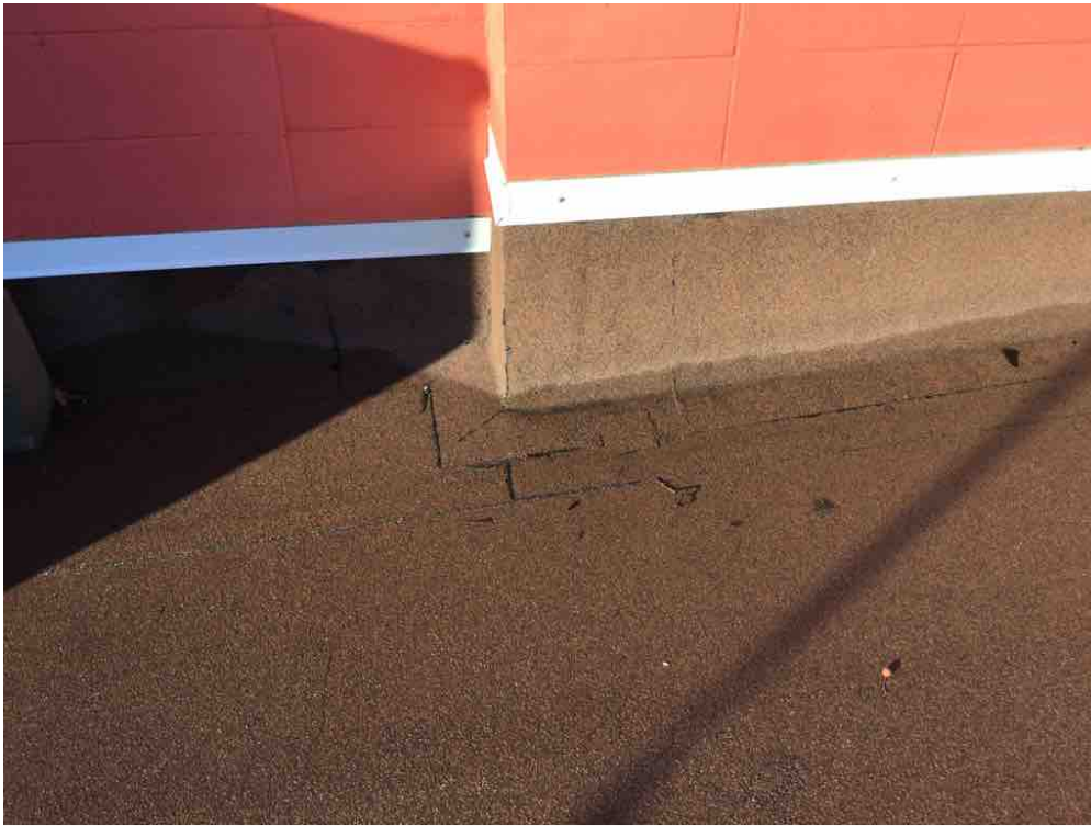
Wall stripping and metal flashings are in good condition.
