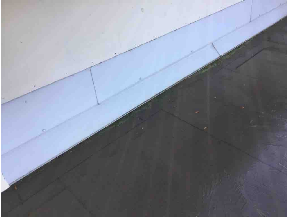
Wall flashing is securely attached and joints are sealed.
