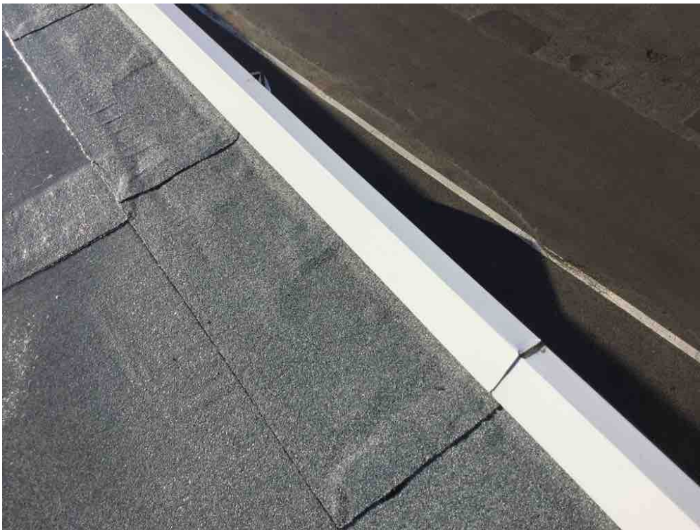
Metal flashings are in excellent condition.
