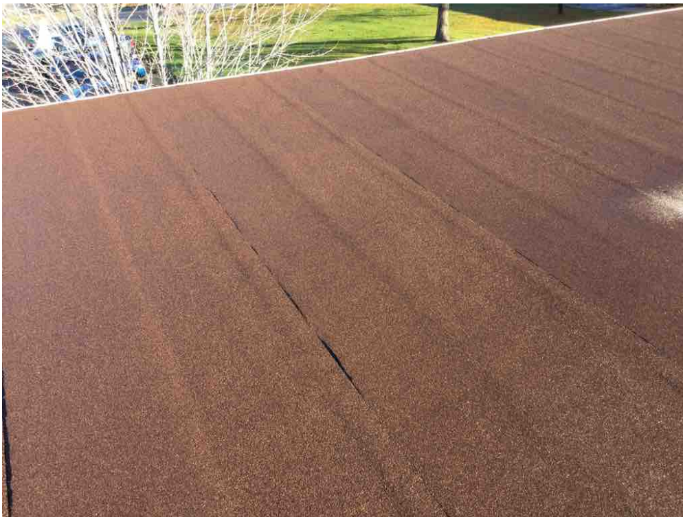
Sloped roof section is in good condition.
