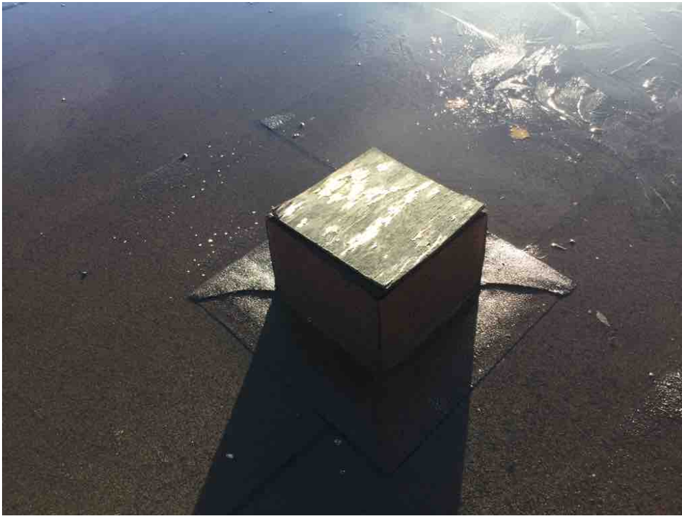
Metal cap should be added.
