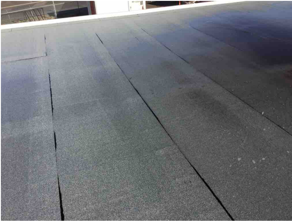
Roof system is relatively new with no membrane application deficiencies noted.
