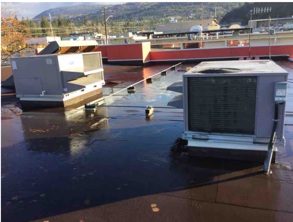
Membrane surrounding air handling units is in good condition.
