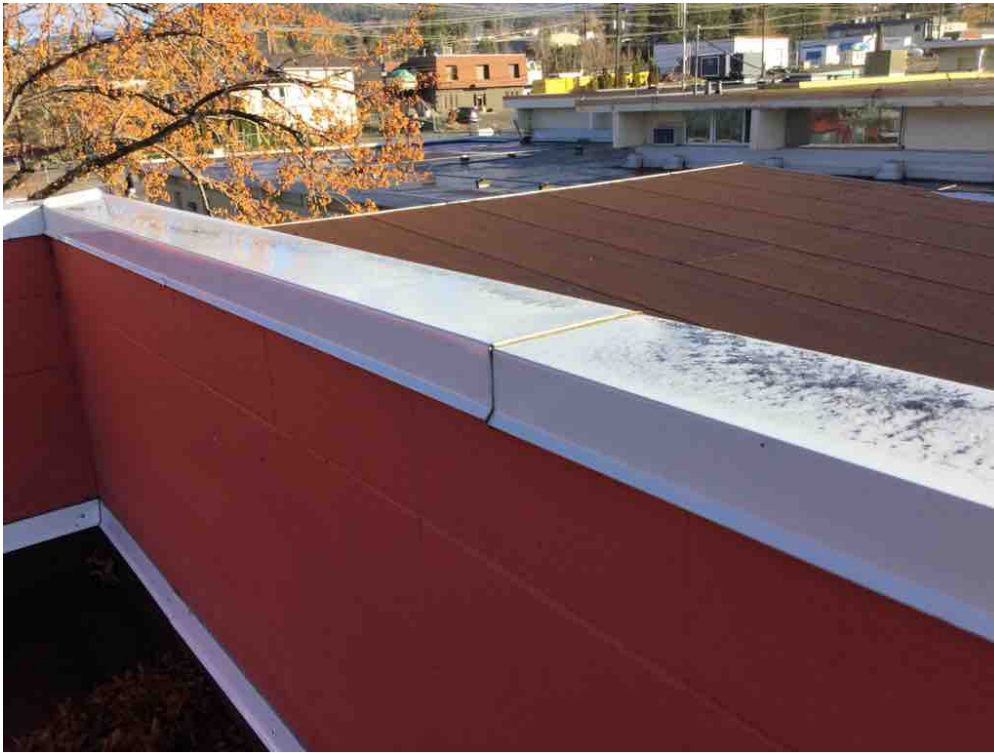
Metal cap flashing is in good condition with all joints sealed.
