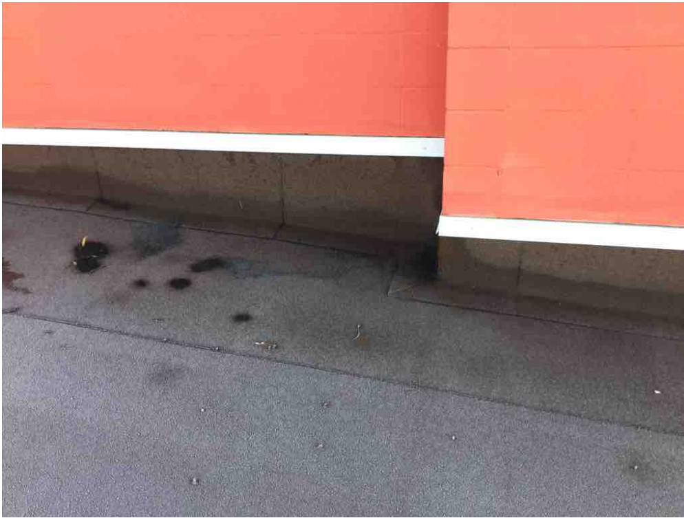
Membrane wall stripping is in good condition .
