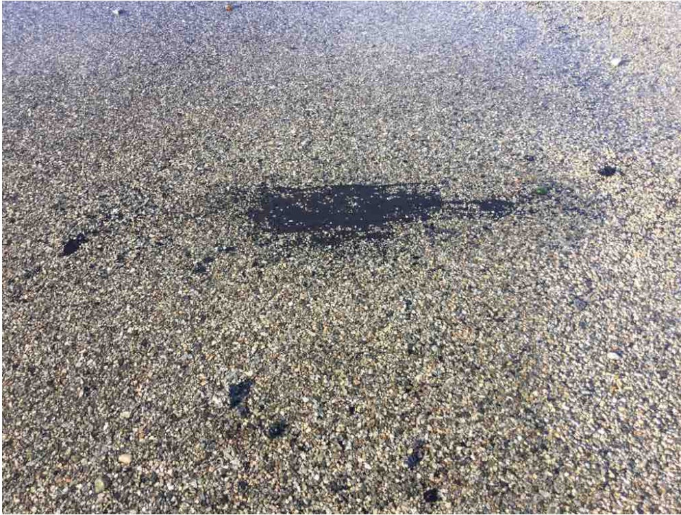
Several repairs have already been completed.
