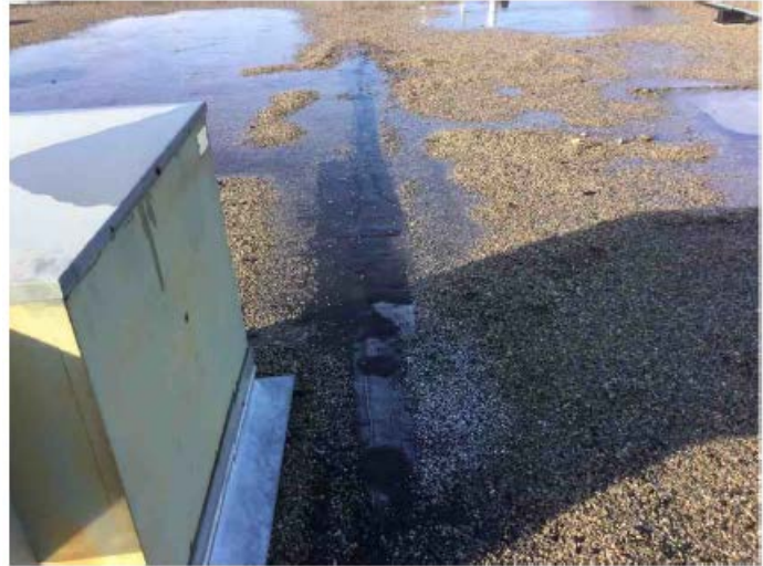
Figure 5. Previous roof repairs
