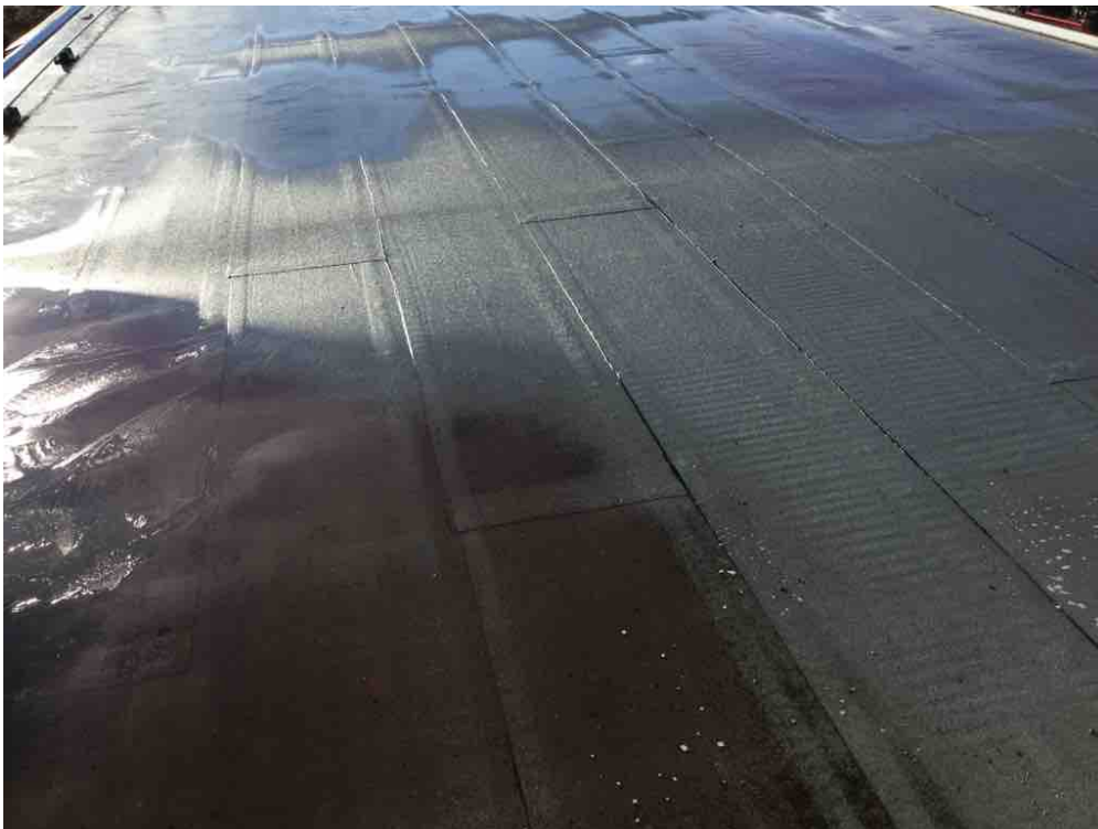
Lower roof section membrane is in excellent condition.
