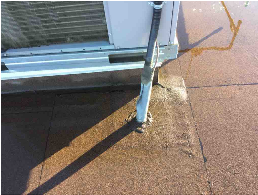
Lead flashing is sealed.
