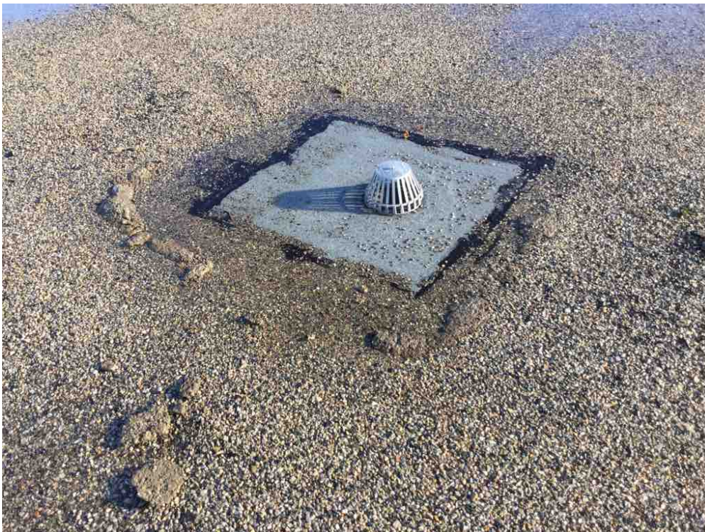
3 New copper spun drains installed.
