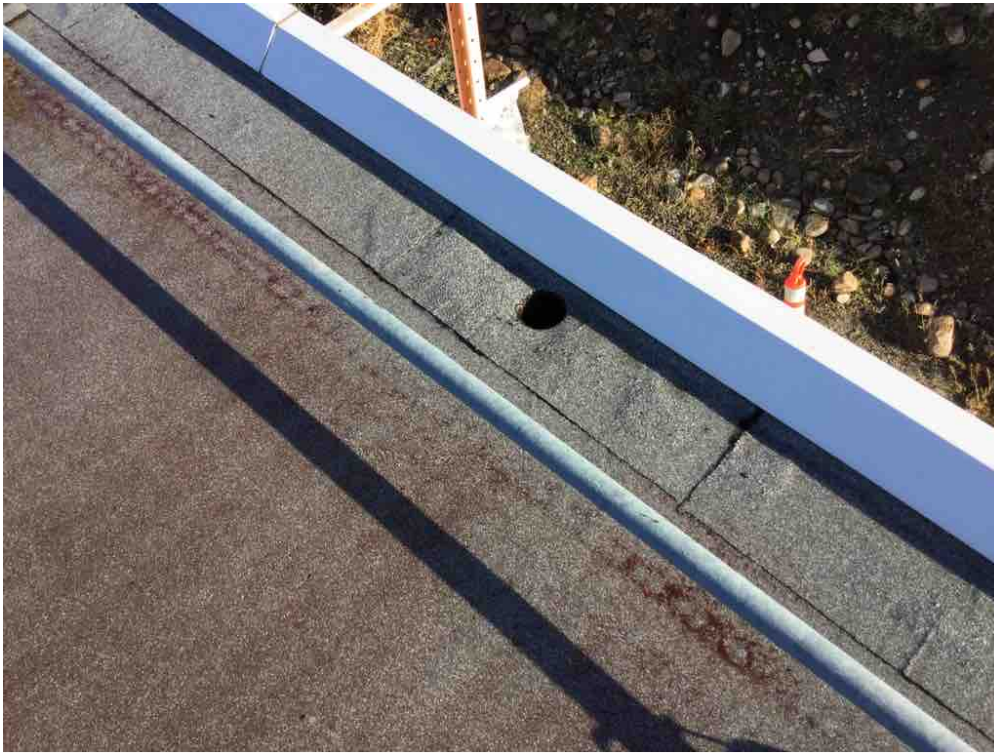
Drains are clear.
