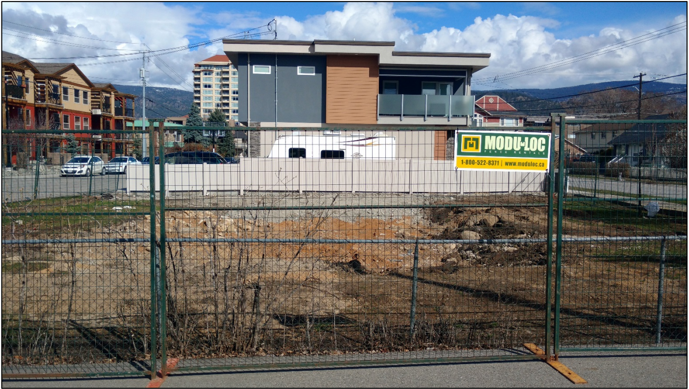
Figure 6: West Elevation (from Walkway)
