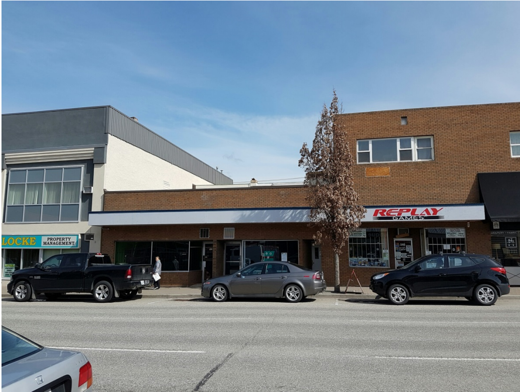
Figure 4: View from Main Street
