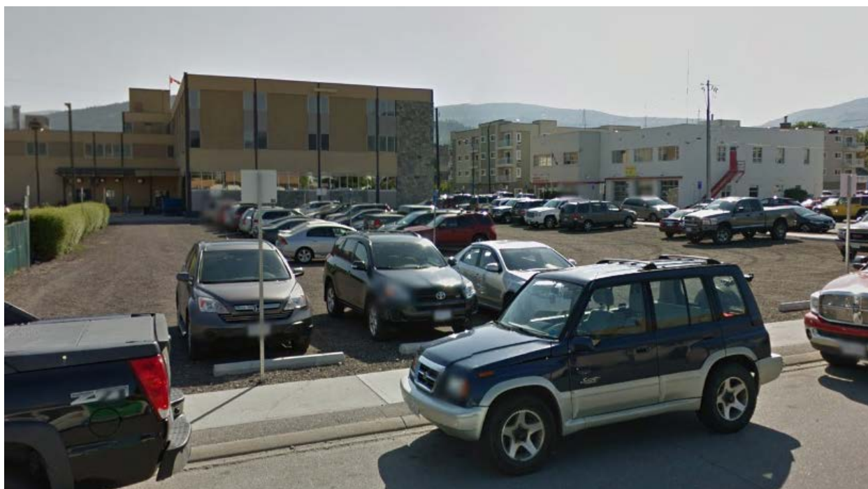
Figure 2: Image of subject property looking east, from Brunswick Street with the CRA building in the mid ground
