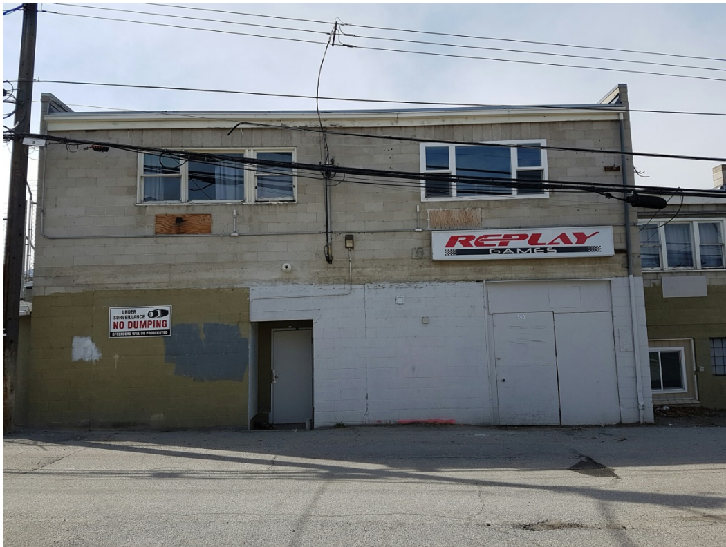
Figure 5: View from the Lane
