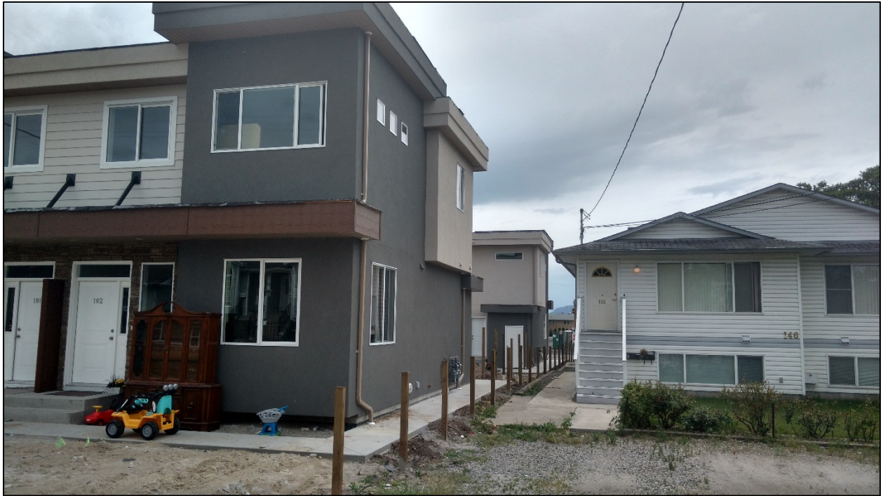
Figure 19: Street view of 134 Cossar Avenue showing proximity to adjacent dwelling
