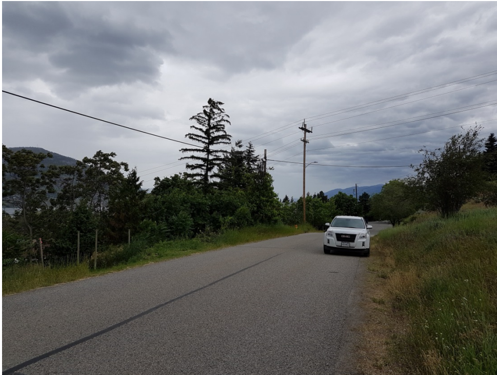
Figure 6: View looking North on Townley street
