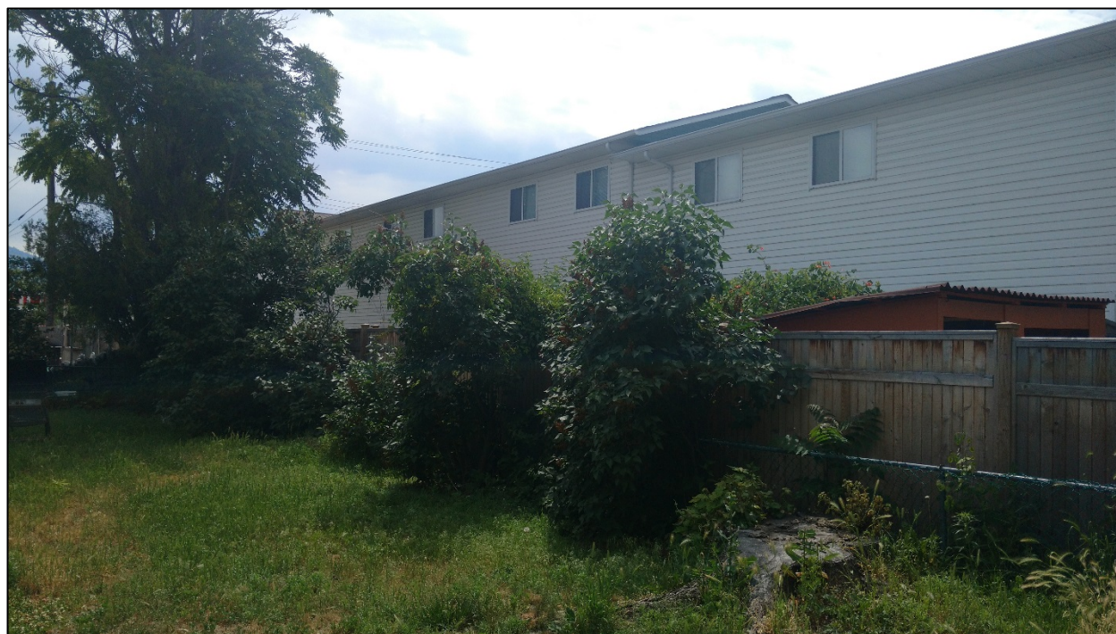
Figure 7: Rear Yard of Subject Property (looking South East)
