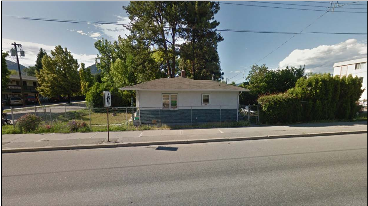
Figure 6: South View (from Westminster Ave West)
