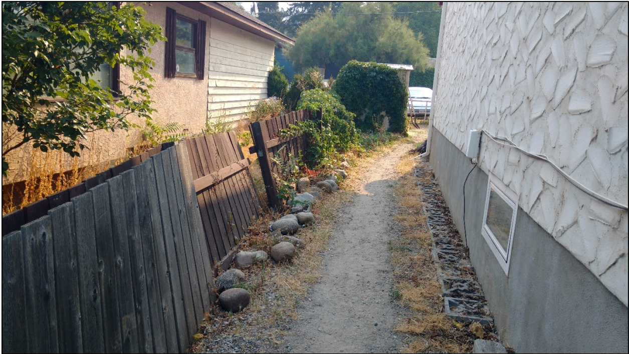
Figure 6: North Side of Existing Duplex with Suite
