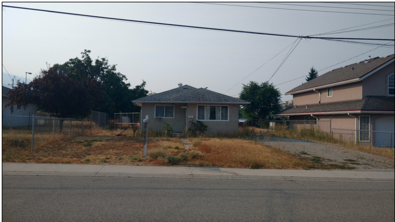
Figure 5: North Elevation of 76 Roy Avenue
