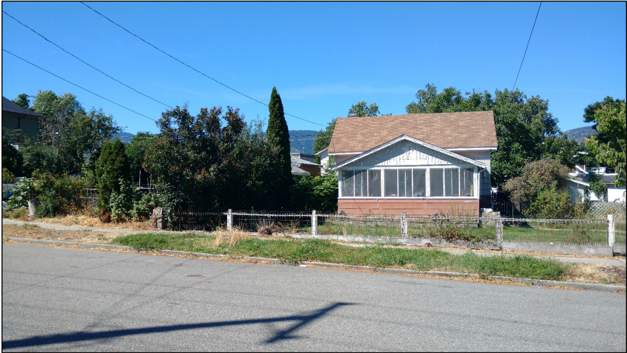
Figure 4: East View (from Papineau St.)
