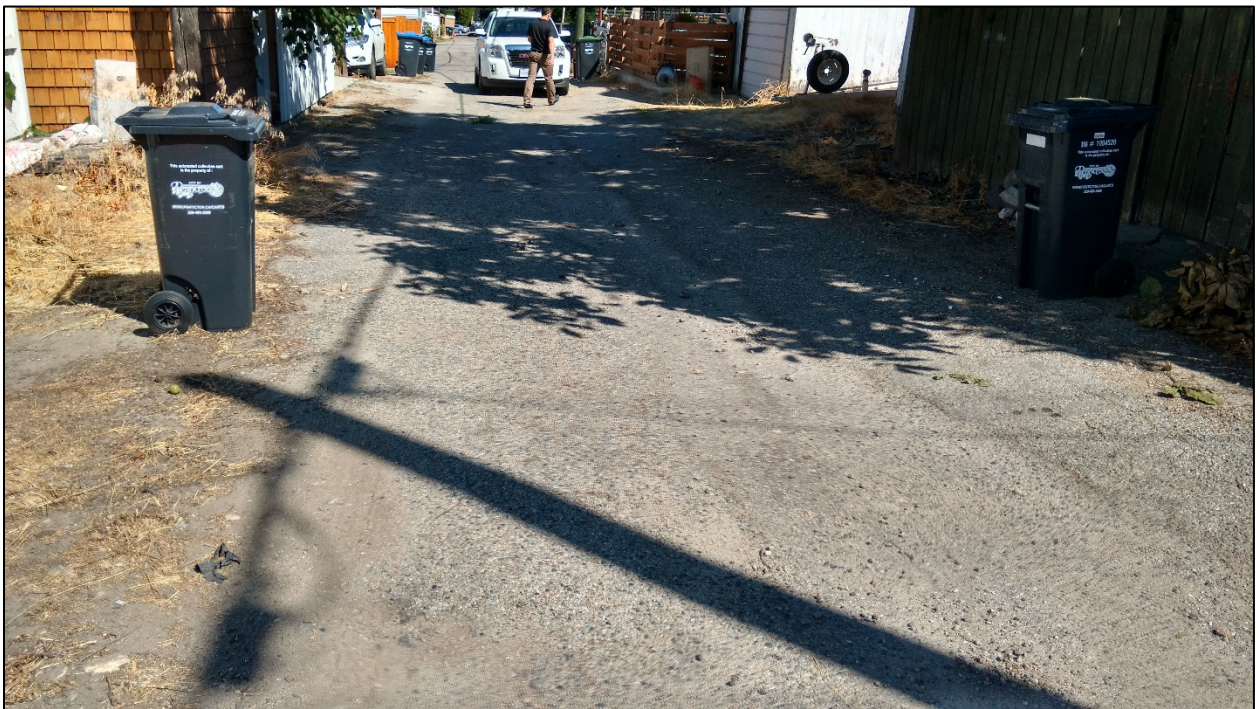
Figure 7: Lane Condition looking North
