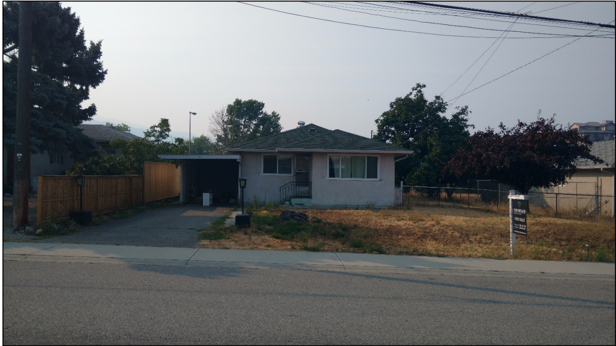
Figure 4: North Elevation of 68 Roy Avenue
