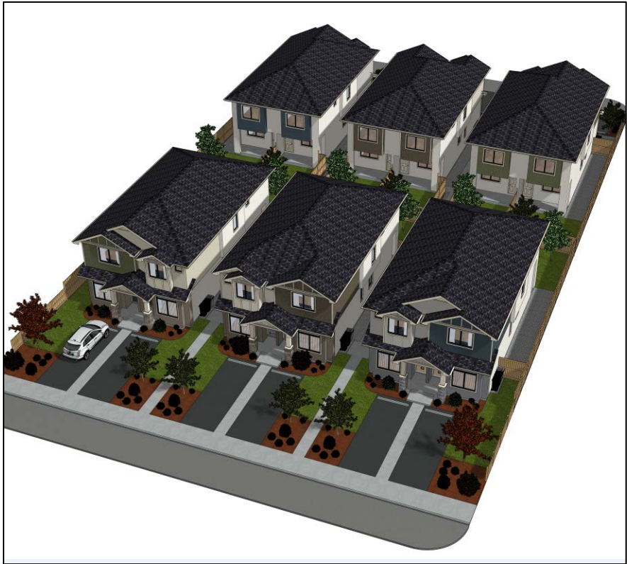
Figure 17: View from Roy Avenue
