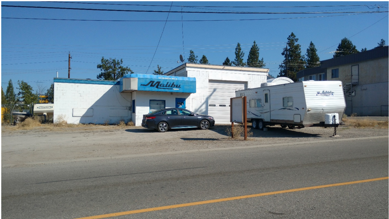
Figure 5: South View of Existing East Building
