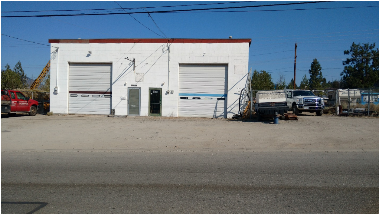
Figure 4: South View of Existing West Building
