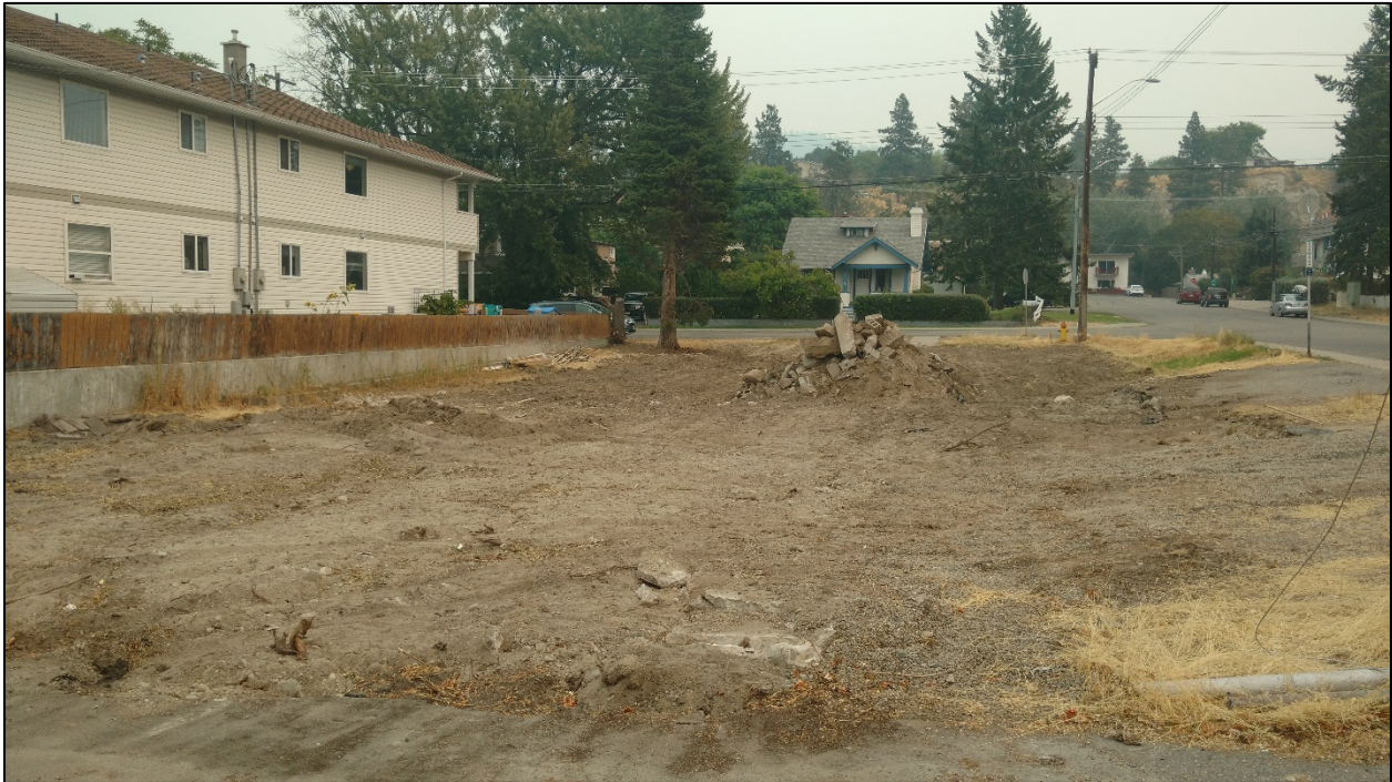
Figure 6: West View (from lane)
