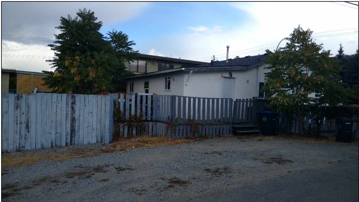
Figure 5: South View (from lane)
