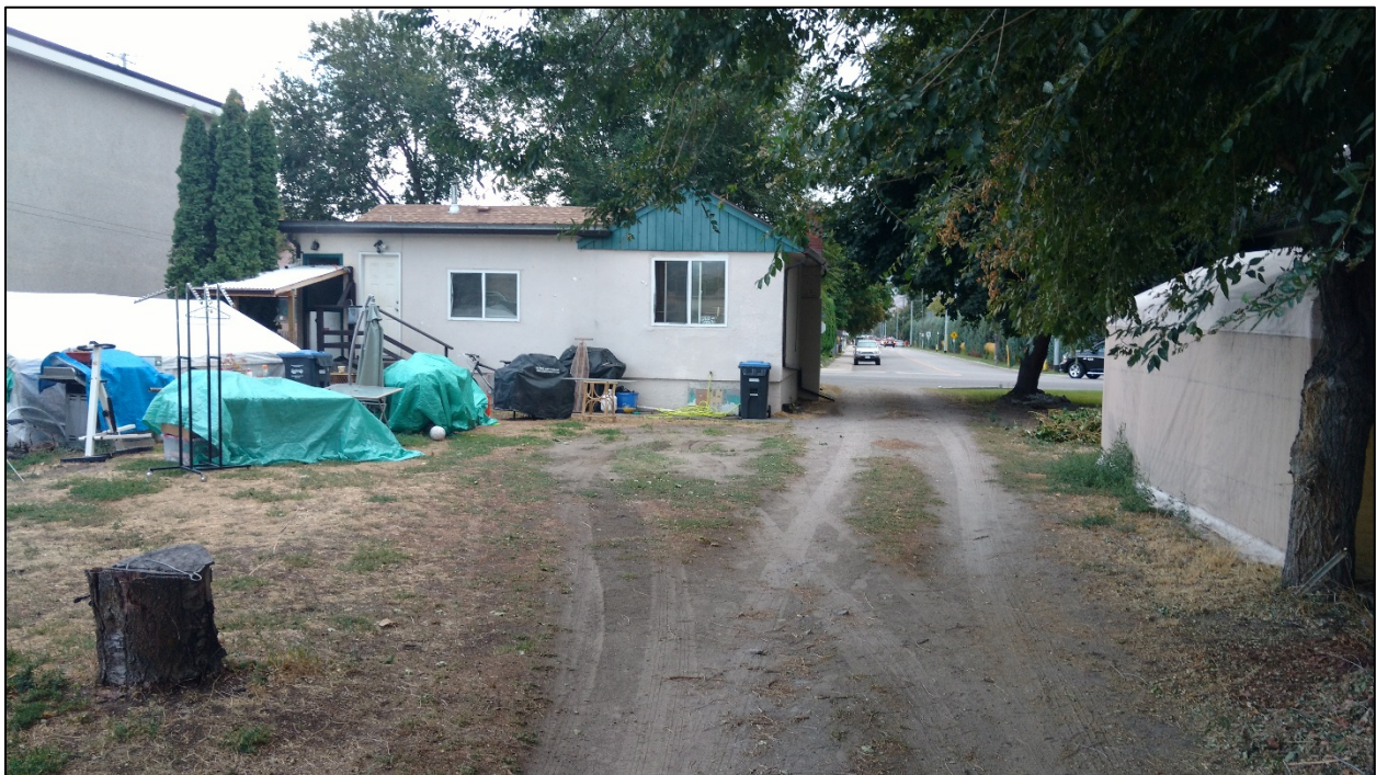
Figure 5: North View (from lane)
