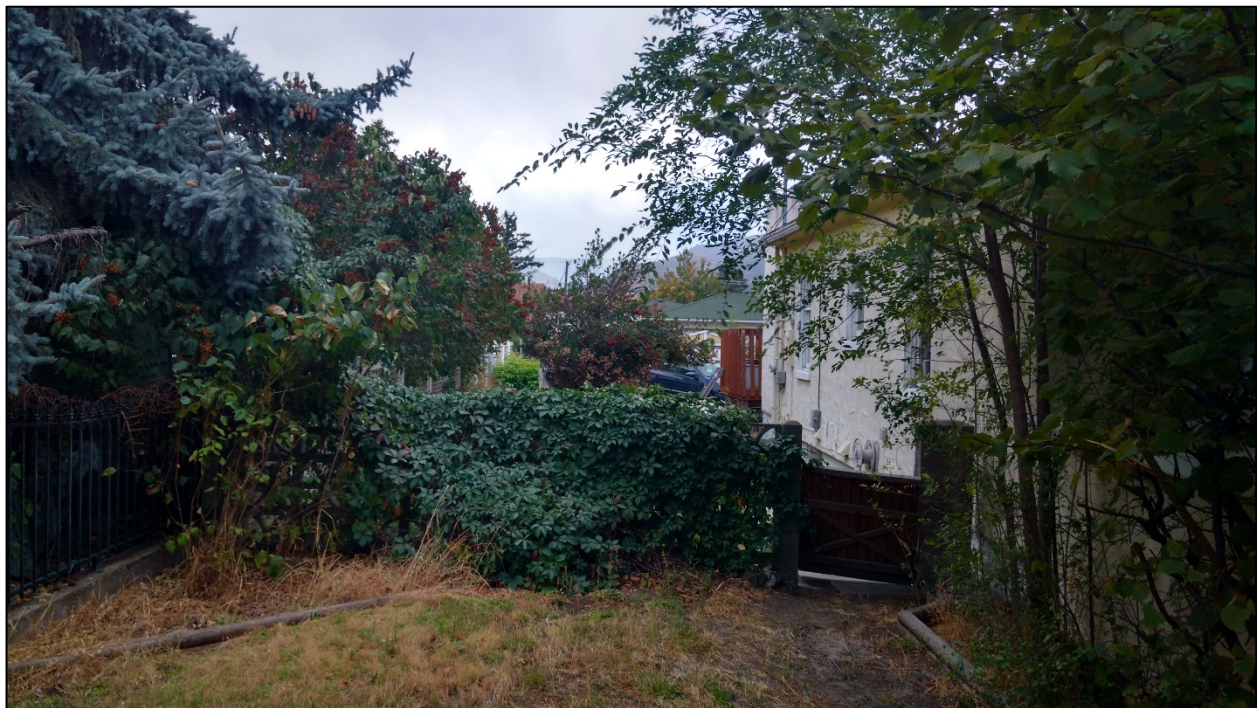
Figure 7: East Elevation showing proximity to neighbours to the south
