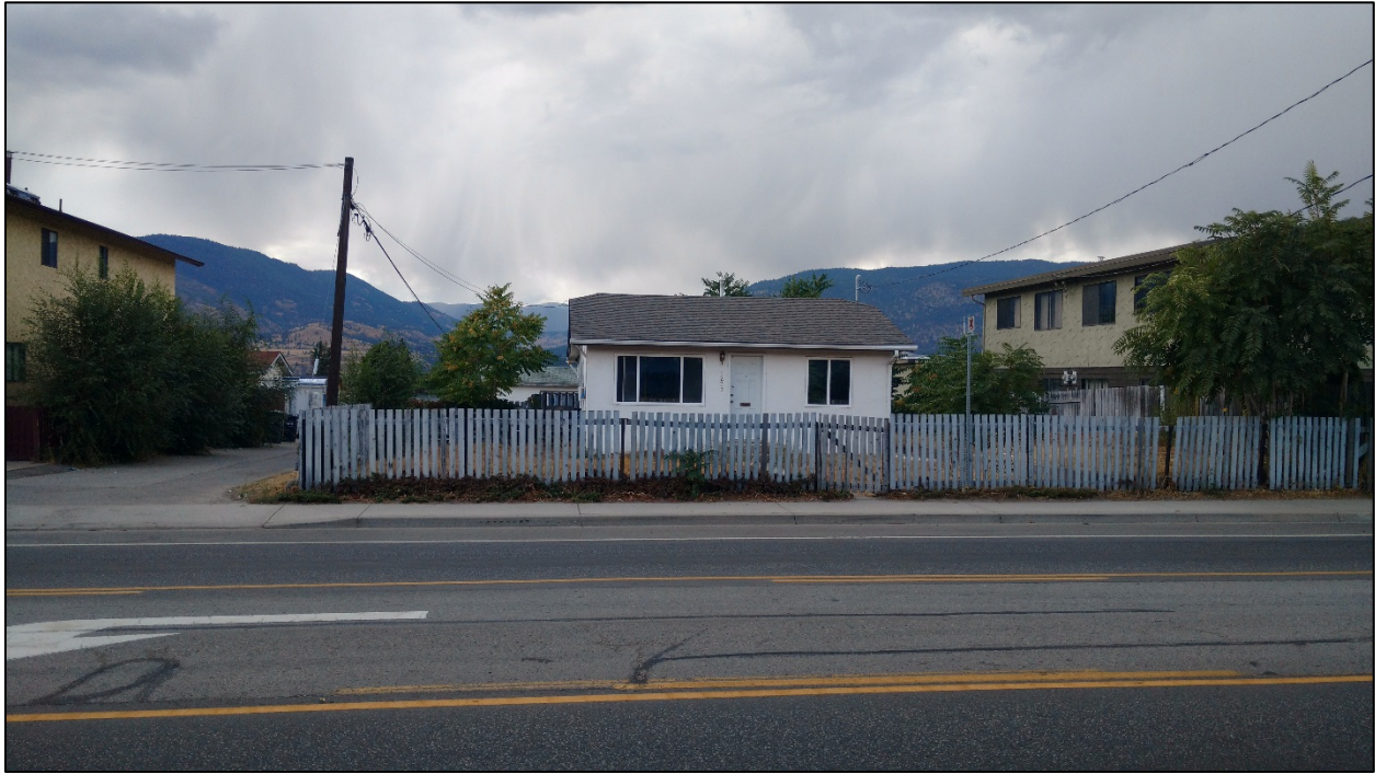
Figure 4: East View of Existing Dwelling (from Government Street)
