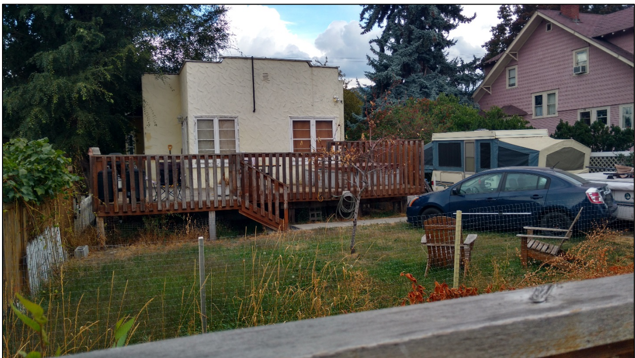
Figure 5: West Elevation (from lane)
