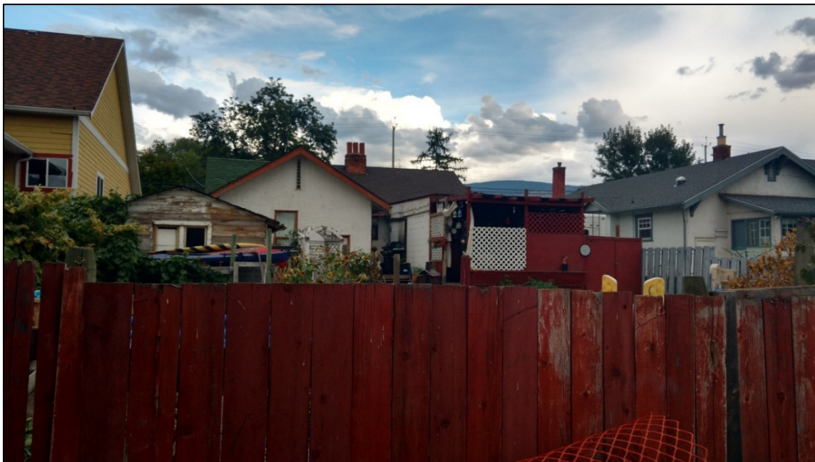
Figure 5: West Elevation (from lane)
