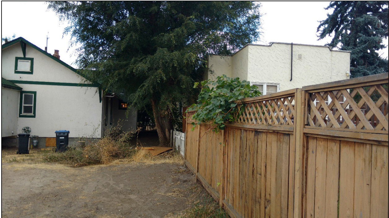
Figure 6: West Elevation showing proximity to neighbours to the North
