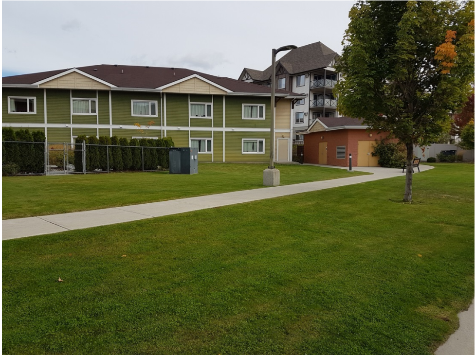
Figure 4: View from Hastings Avenue
