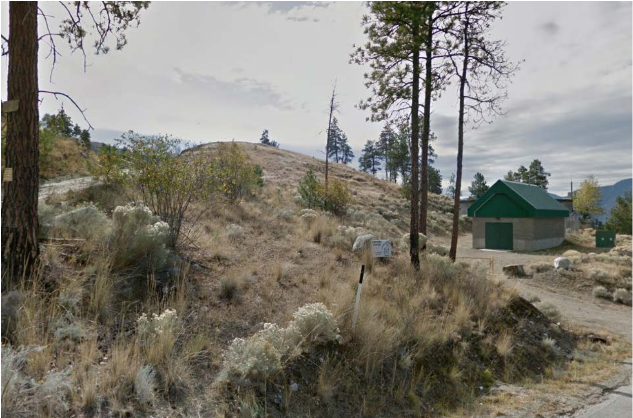
Figure 3: Image of subject lands looking west with water pump house in mid-ground
