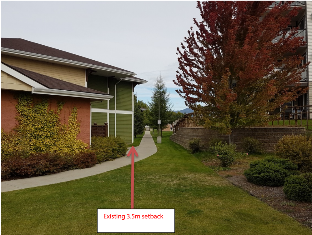
Figure 5: View from Hastings Avenue
