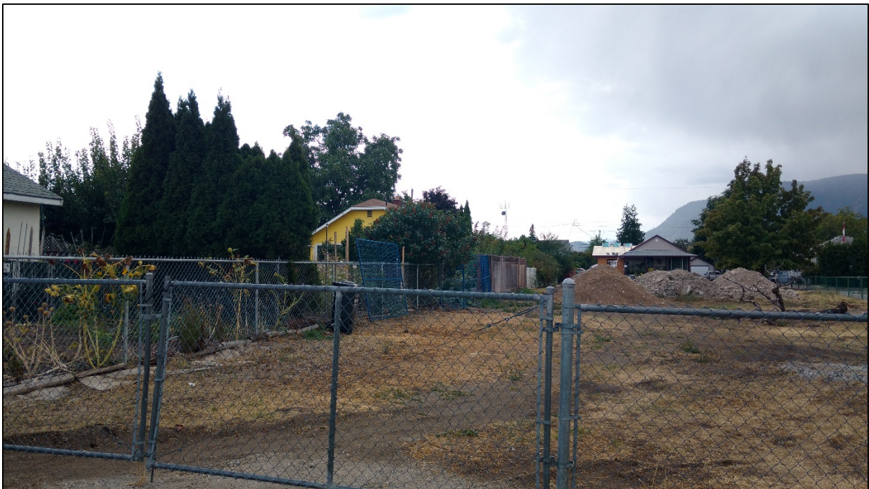
Figure 7: North View looking towards the east neighbour
