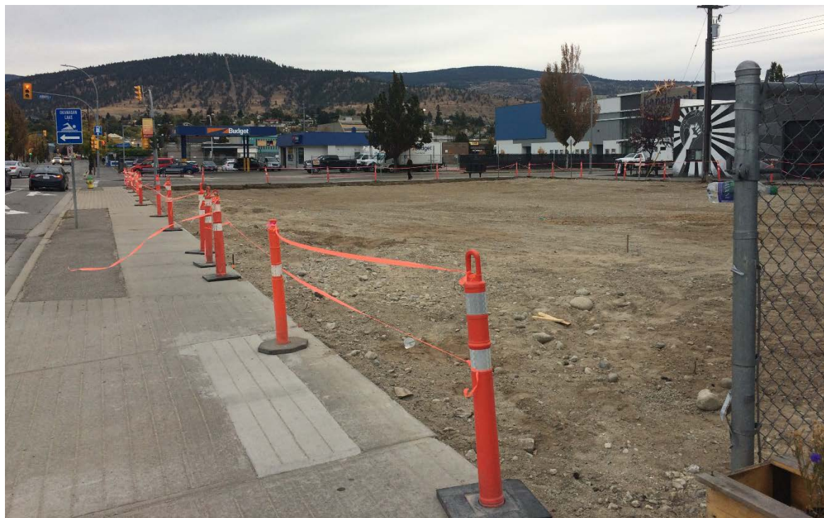
Figure 2: Frontage of subject property along Westminster Avenue showing the existing curb returns
