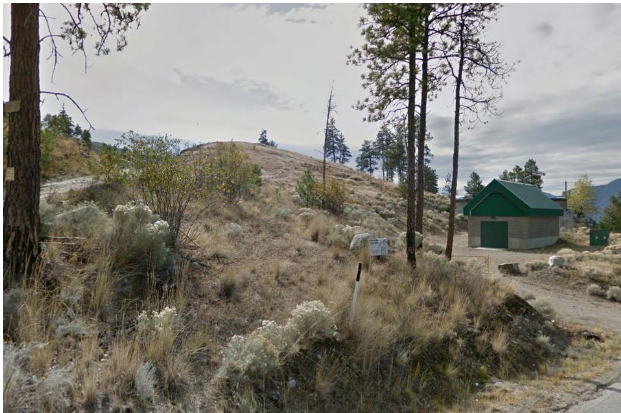
Figure 3: Image of subject lands looking west with water pump house in mid-ground
