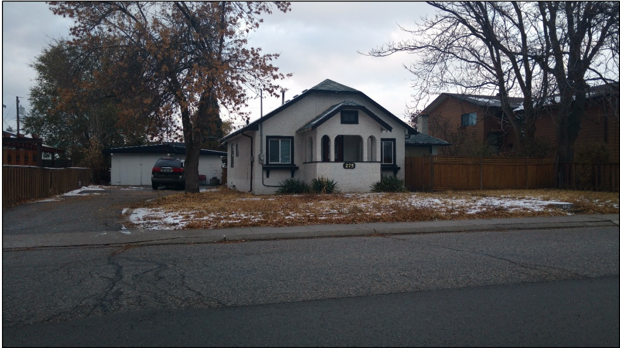
Figure 4: South View of Subject Property (from Conklin Avenue)
