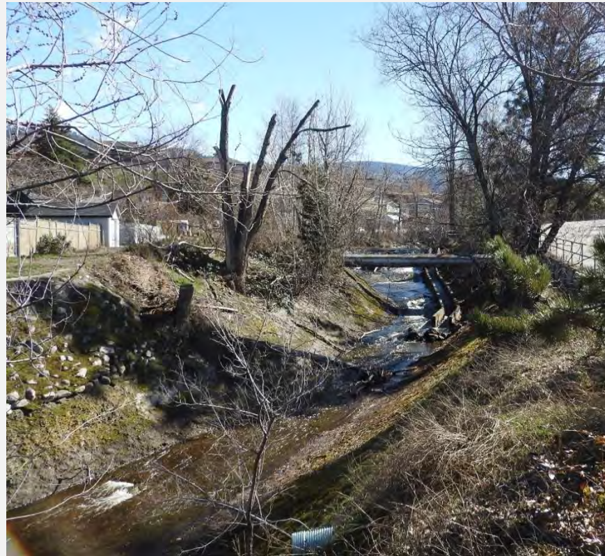
Looking upstream at the aboveground sewer crossing and Structure #3
