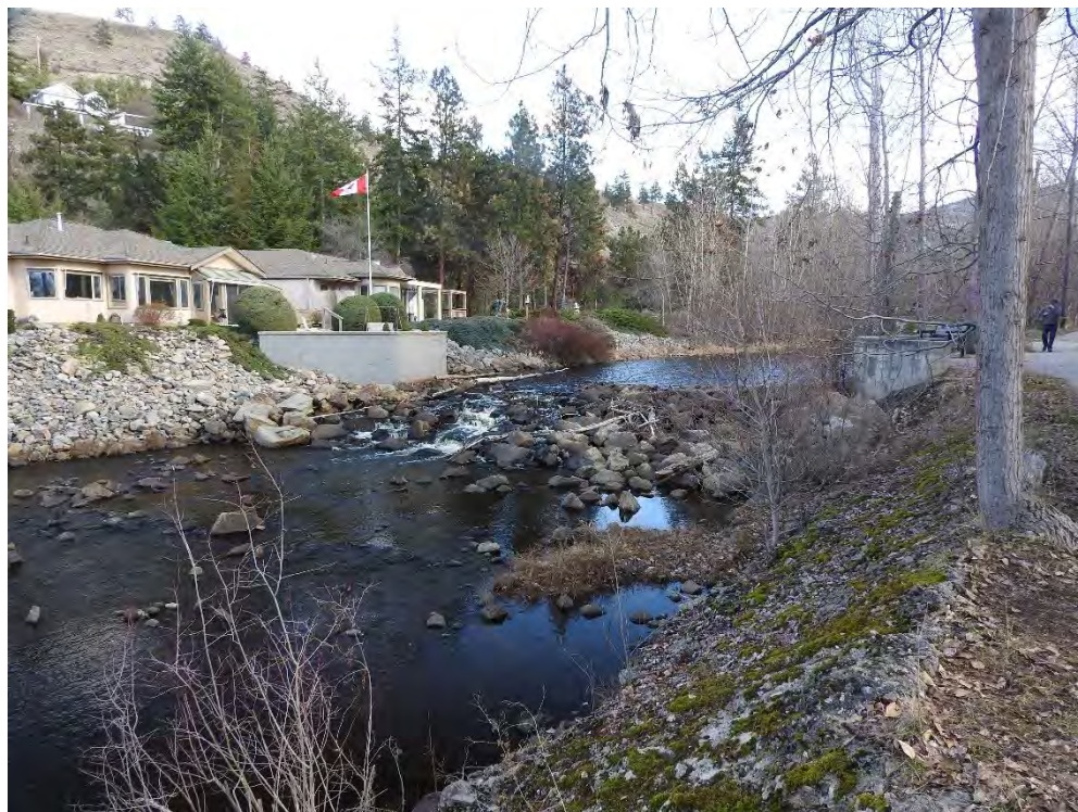
Drop Structure with Riprap Apron
