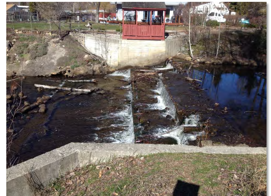
Wood Crib Drop Structure with Rock and Concrete
