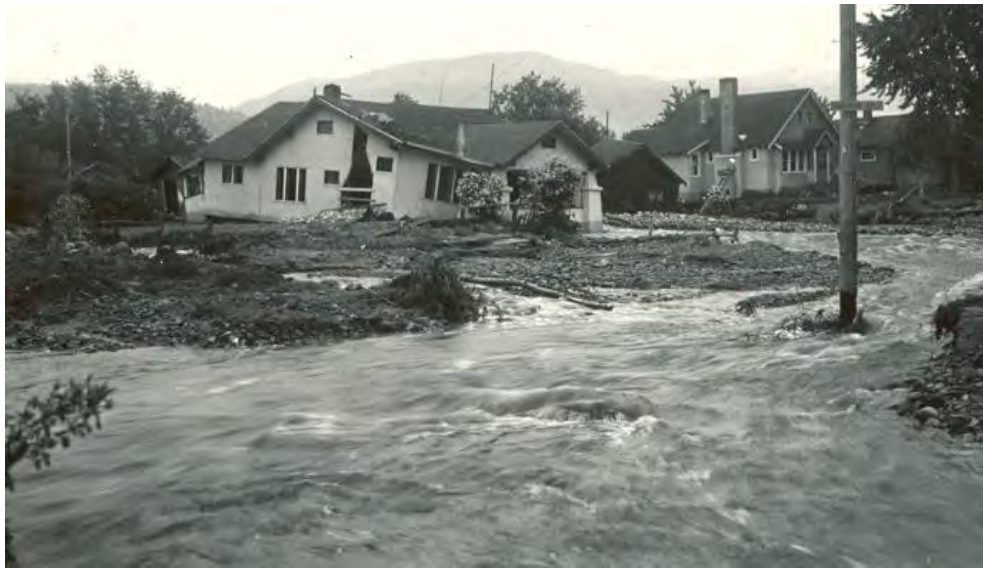
Flooding damage at Van Horne St. & Nanaimo Ave. (Source Unknown, 1942)
