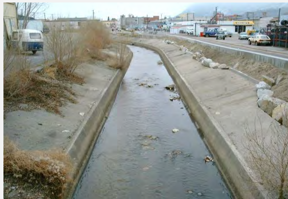
Formed concrete lining, facing upstream
