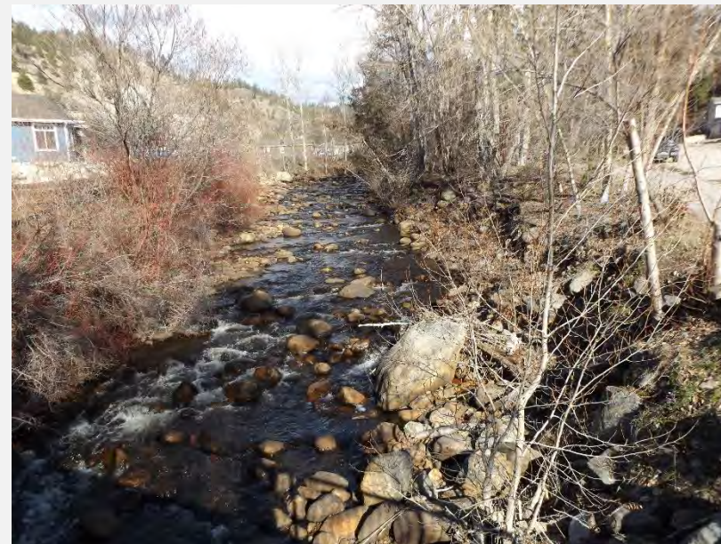
Looking upstream at Reach 13
