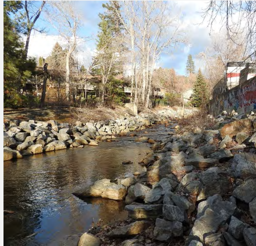
Looking upstream at Reach 9
