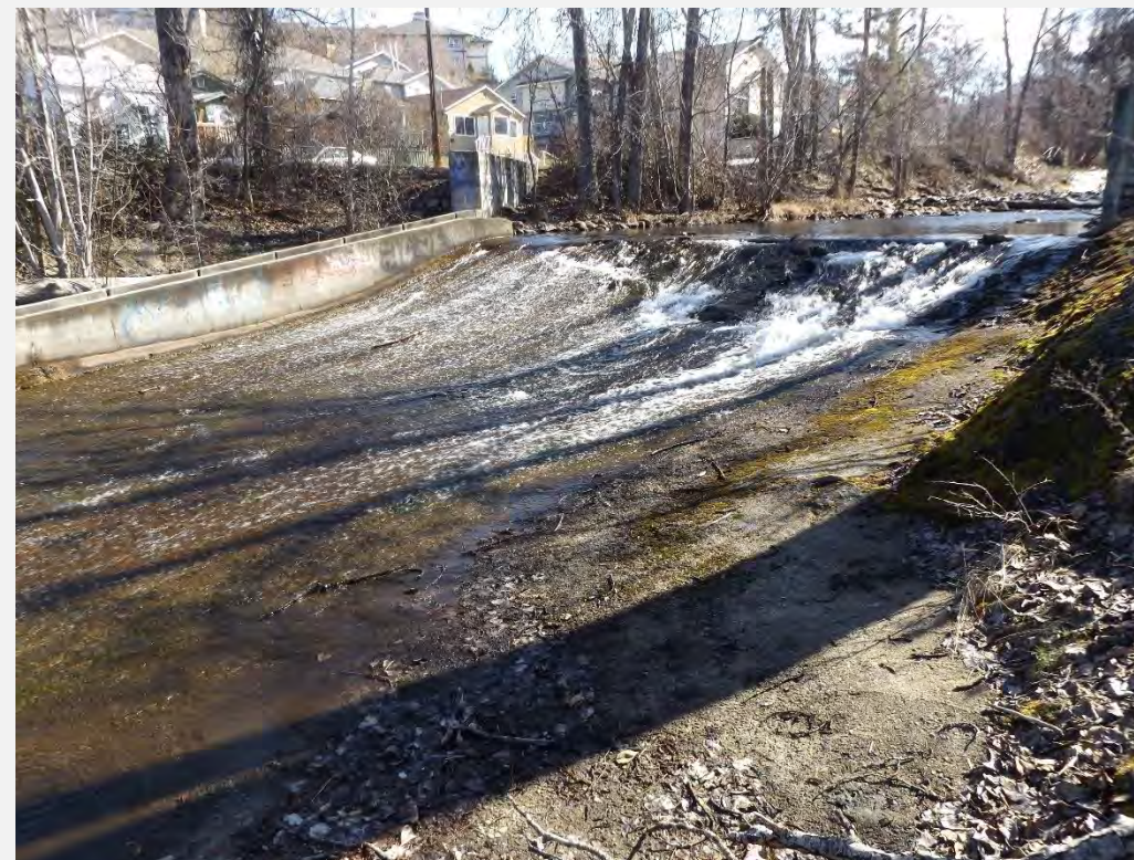
Looking upstream at the concrete crest and apron of Structure #4
