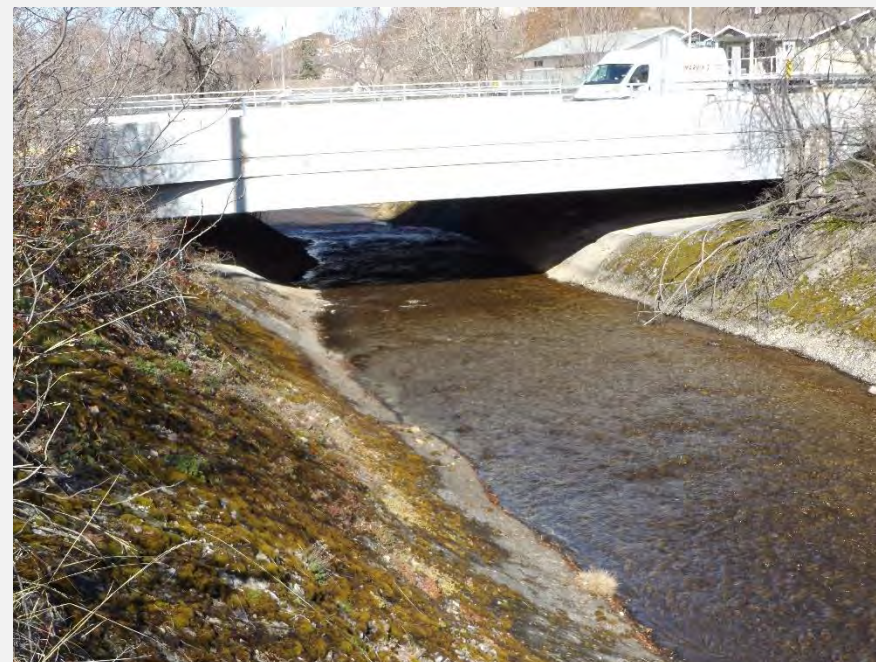
Looking downstream at Eckhardt Avenue bridge
