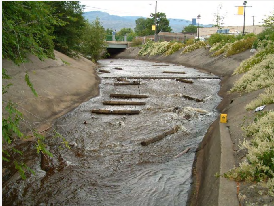
Looking upstream at Structure #1
