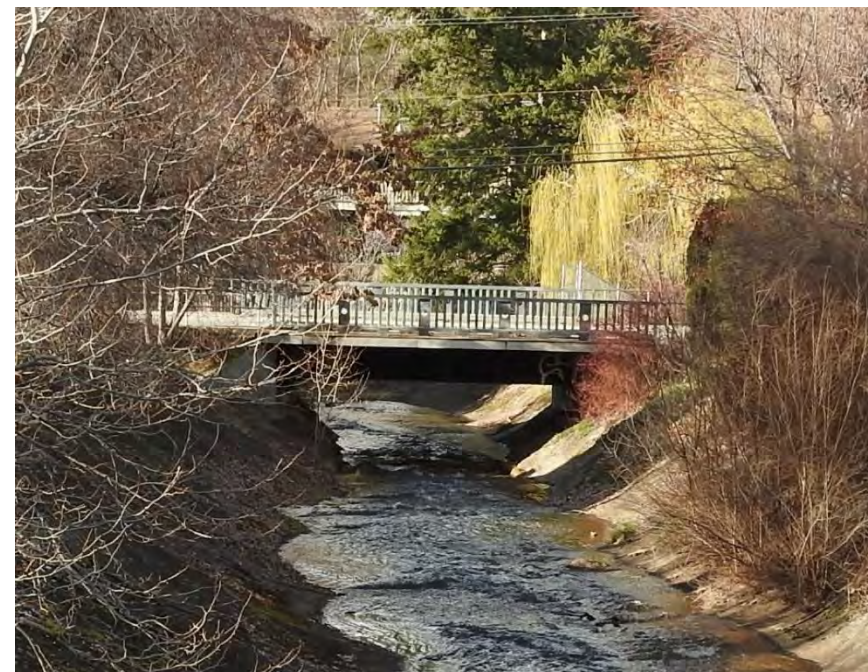
Channel Narrowing at Forestbrook Drive bridge
