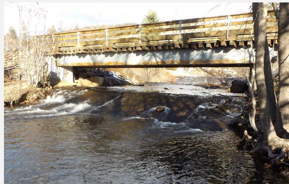
View of McNicoll pedestrian bridge and Structure #26 from downstream
