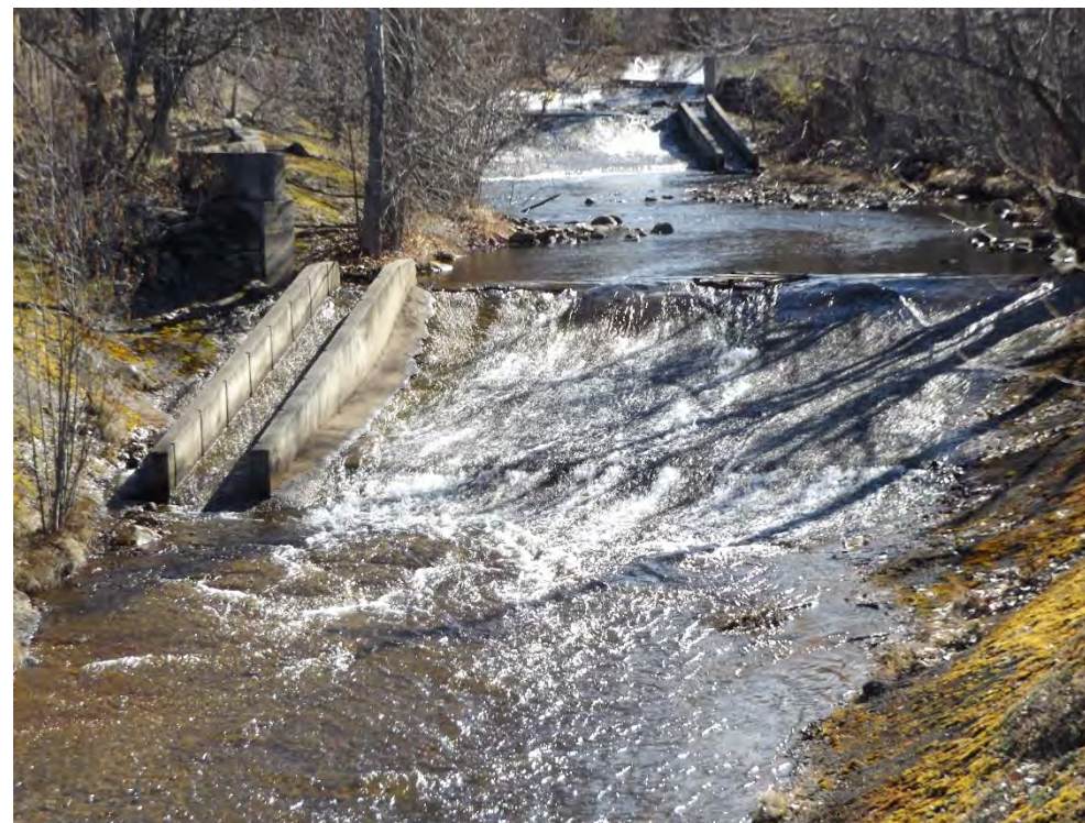
Drop Structure with Concrete Crest and Apron
