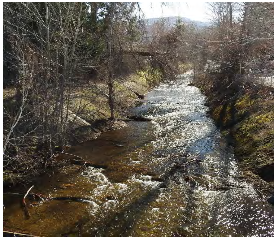
Section 1 – Concrete Lined
