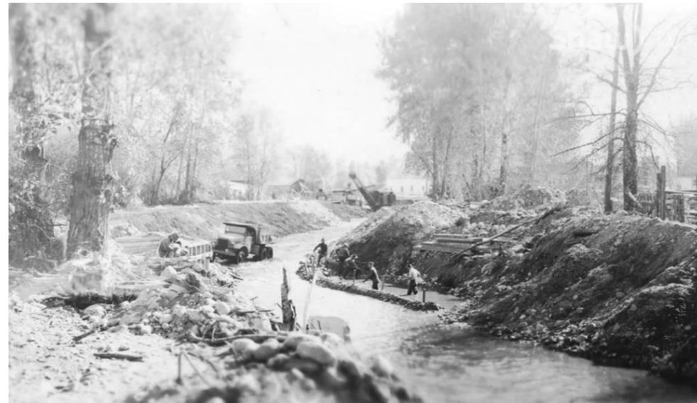
Construction of concrete lining. (Source Unknown)
