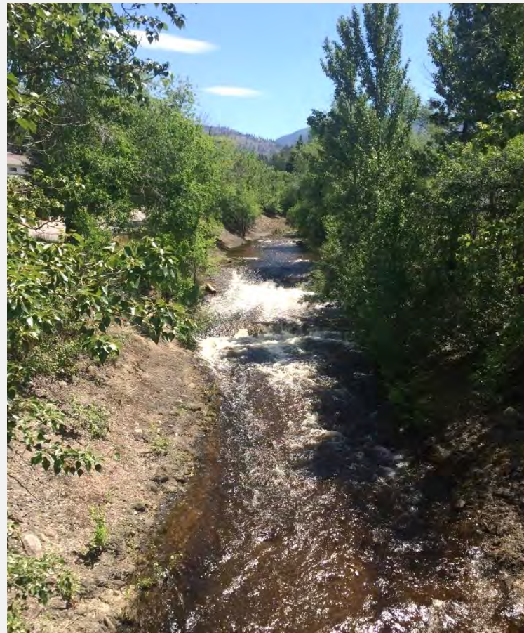
Looking upstream at Structure #6, from the KVR pedestrian bridge
