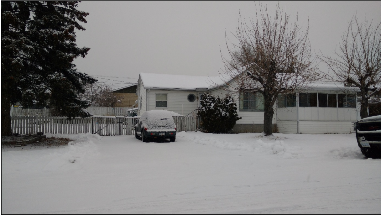
Figure 4: South View (from Phoenix Avenue)
