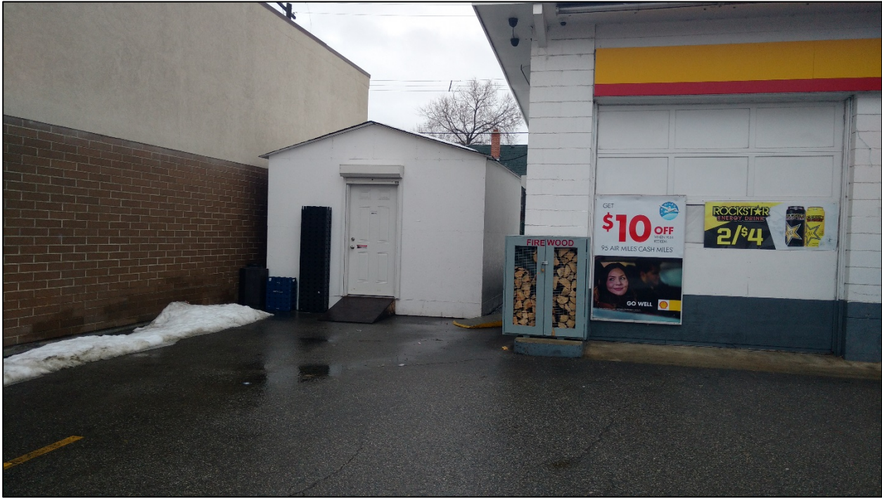
Figure 5: West Elevation of existing gas station and shed
