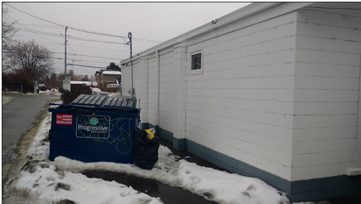
Figure 6: East Elevation from the lane looking south
