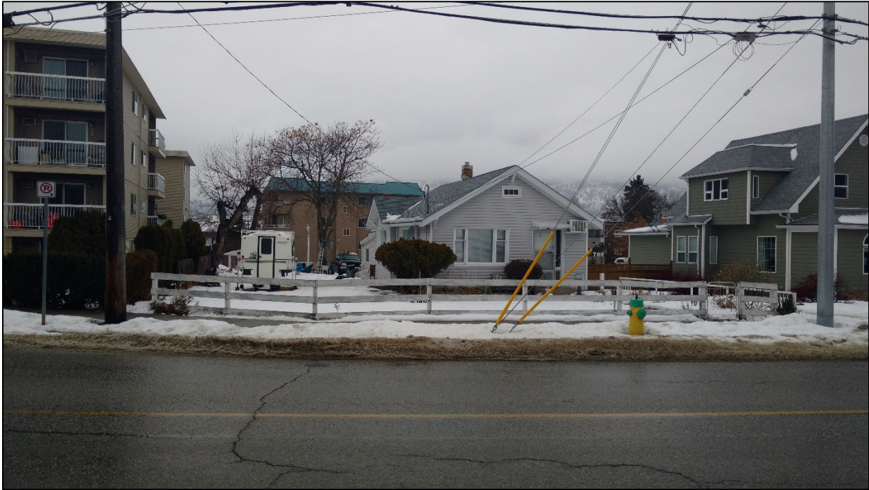
Figure 4: East View of subject property (from Martin Street)
