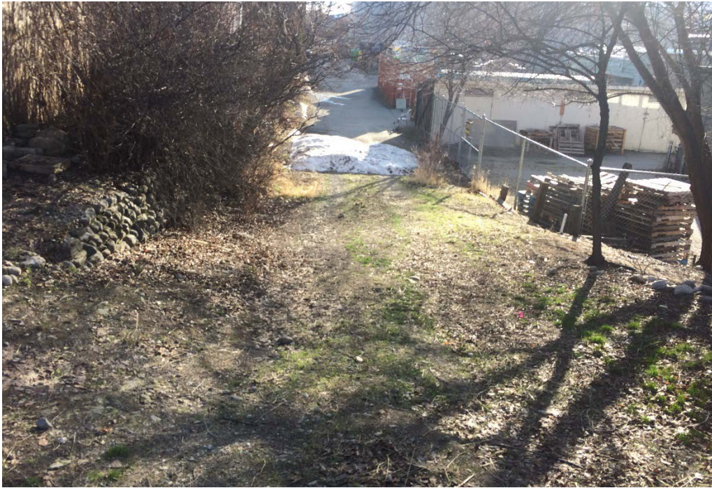
Figure 4: Image of unconstructed back lane looking towards paved portion of the lane (south)
