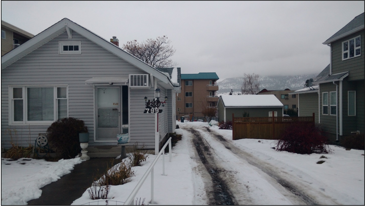
Figure 7: East View showing proximity to neighbouring property to the north
