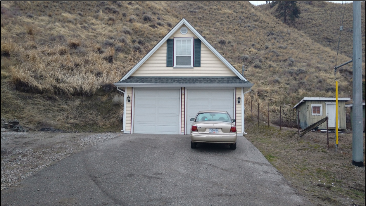
Figure 4: West View of Existing Garage (to be demolished)
