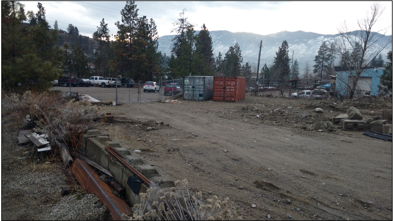
Figure 6: North View of Subject Property
