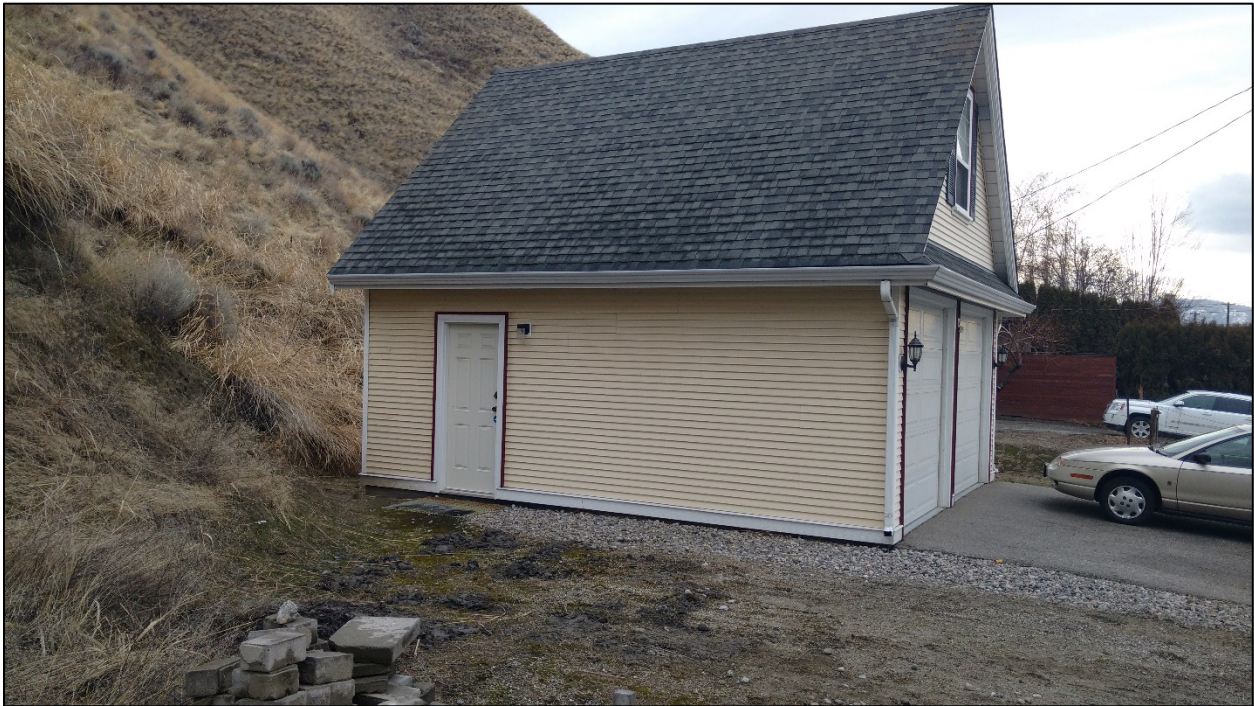
Figure 5: North View of Existing Garage
