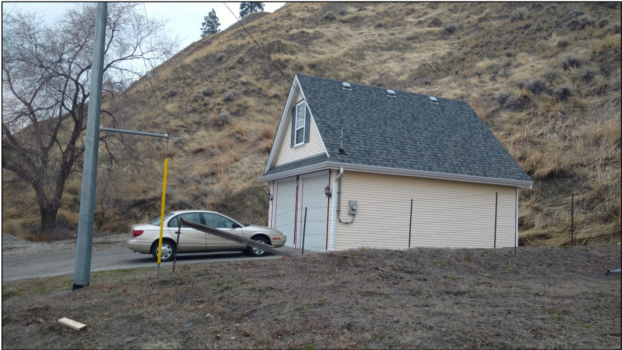
Figure 6: South View of Existing Garage
