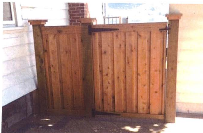
Treated post set in concrete Cedar fence boards and rails
