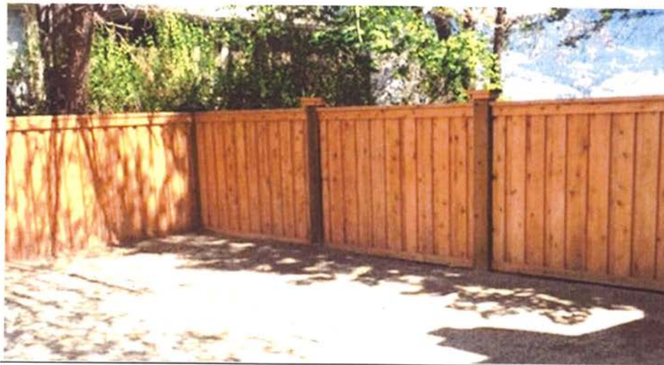
Treated post set in concrete Cedar fence boards and rails
