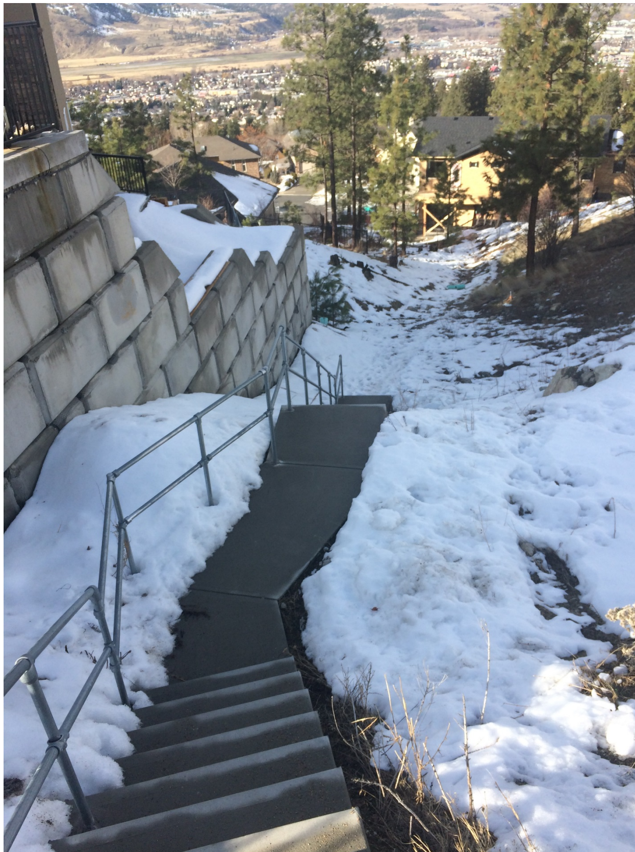
Figure 1: Image of public walkway looking west with existing over-height retaining wall on left. Similar wall is proposed on right.
