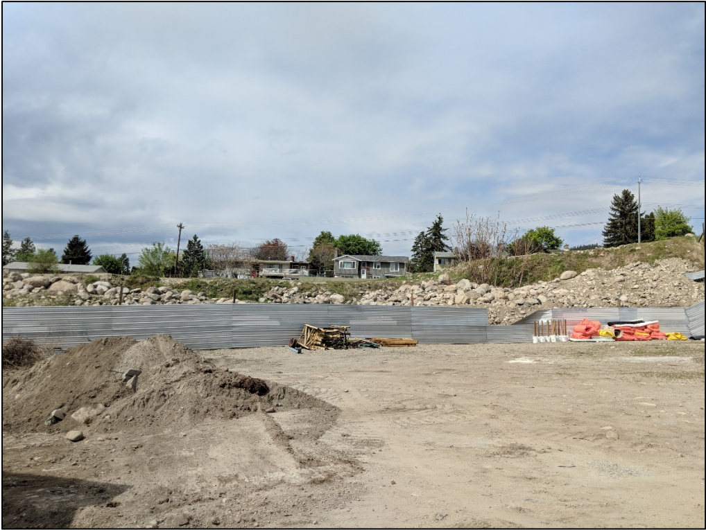
Figure 9: Rear Portion of Proposed Lot B (looking North)
