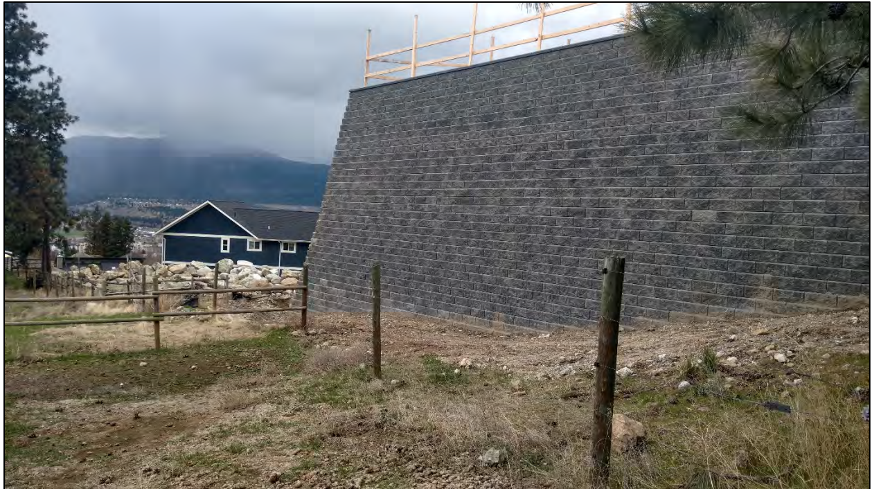
Figure 6: South Elevation looking west
