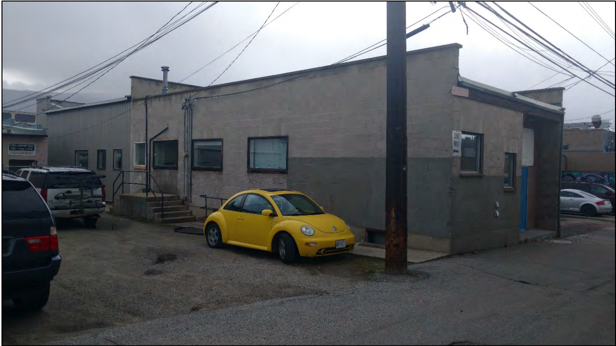
Figure 6: South View (from the lane)
