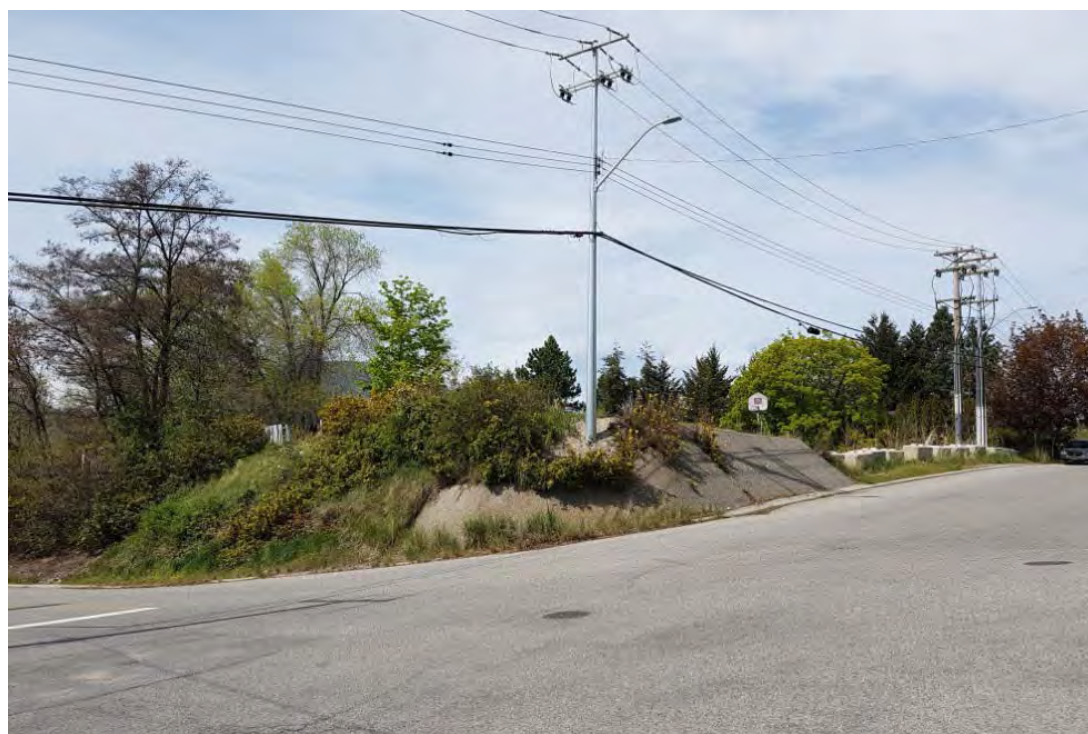
Figure 7: View at the corner of Westminster Avenue and Abbott Street, as part of the project the overhead lines would be undergrounded at the cost of the developer.
