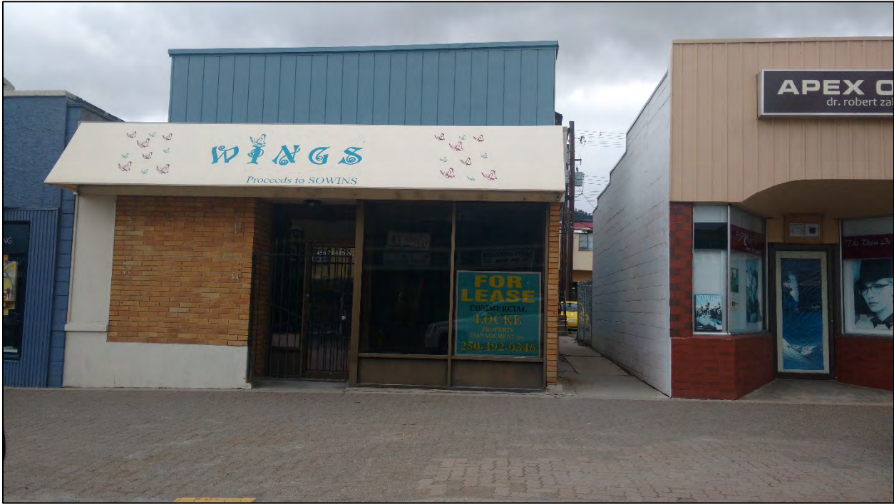
Figure 4: West View (from Main Street)
