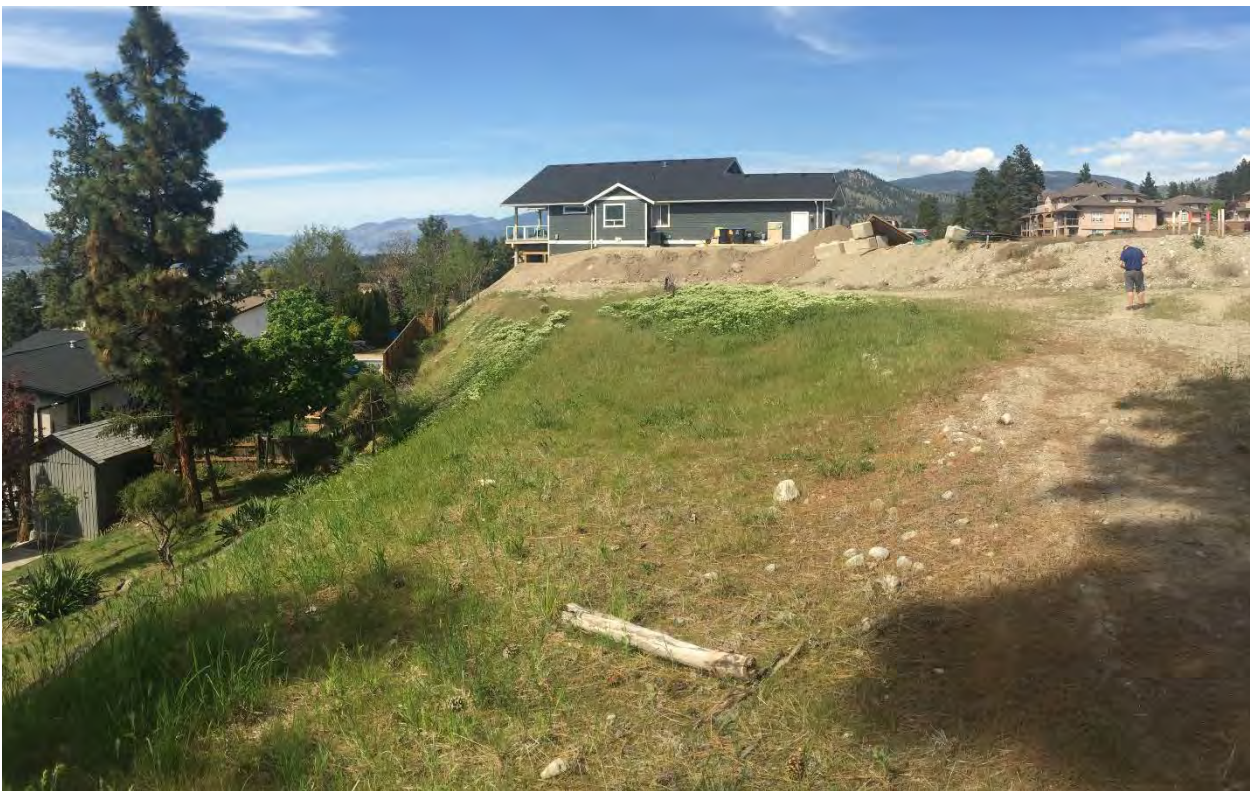
Figure 4: Properties along Timberstone Place looking down on Laurel Place
