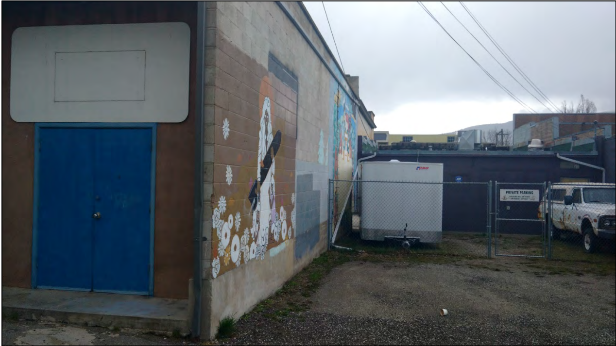
Figure 7: North Building Face (from the lane)
