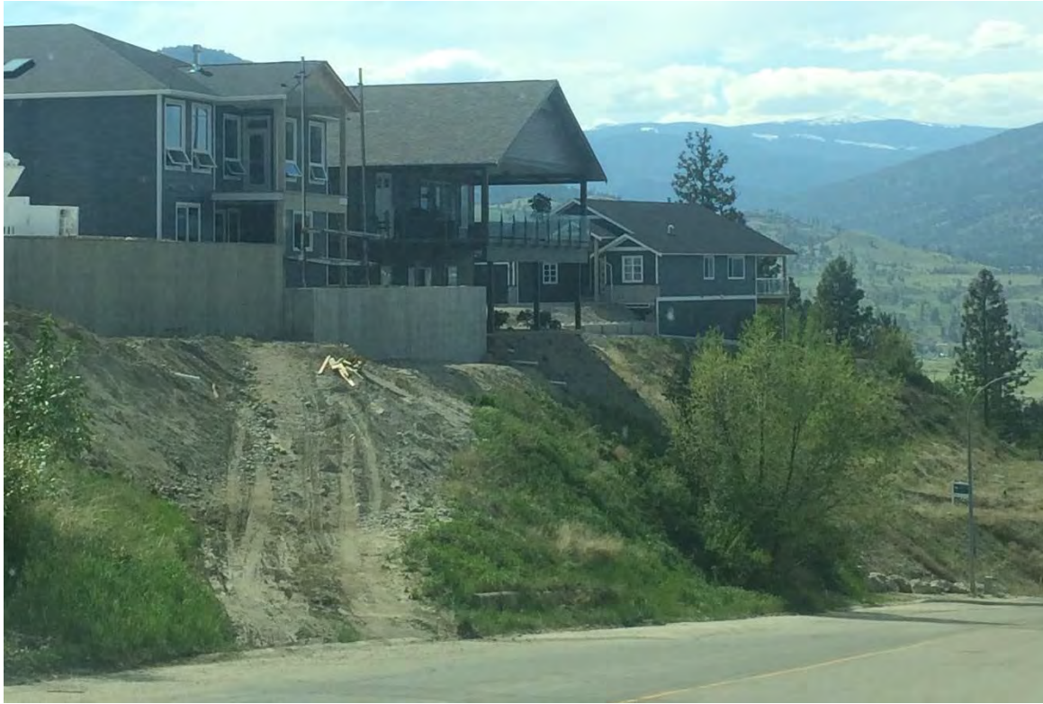
Figure 1: Area along Balsam Avenue where retaining walls are proposed
