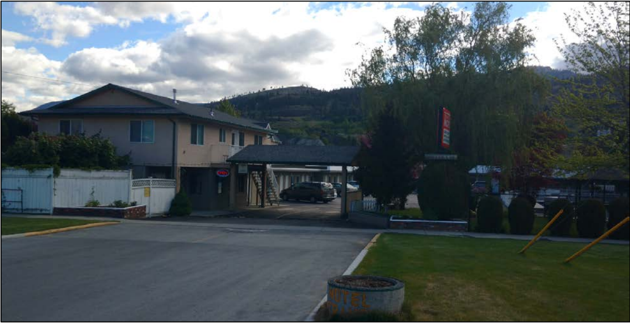
Figure 4: West View of Subject Property (from Skaha Lake Road)
