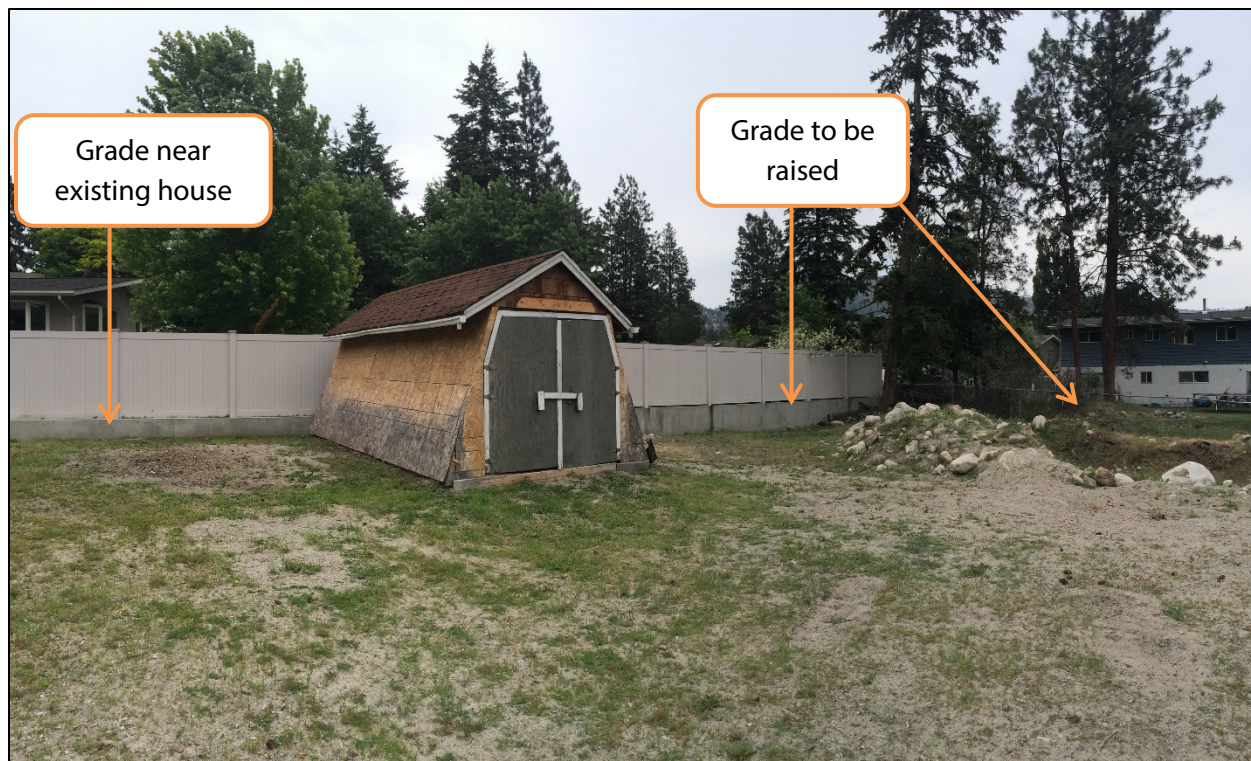
Figure 9 – Backyard to be re-graded to maintain same grade across the backyard
