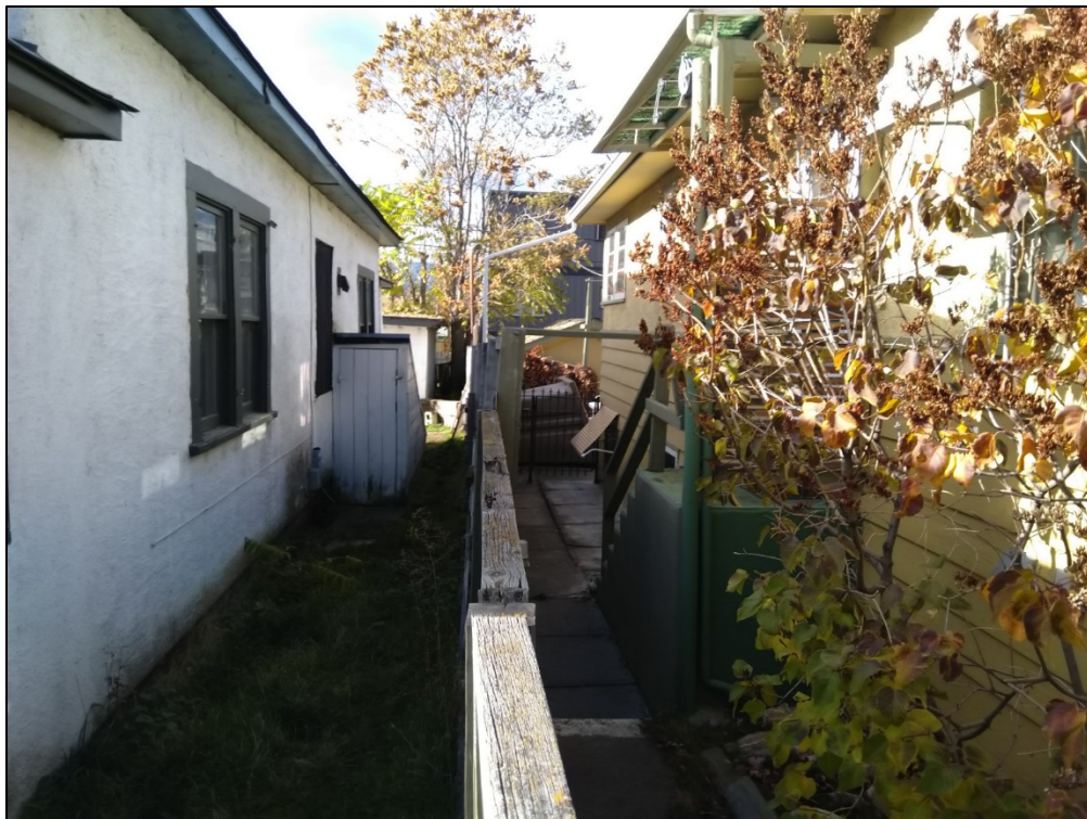
Figure 7: East View showing proximity to north neighbour
