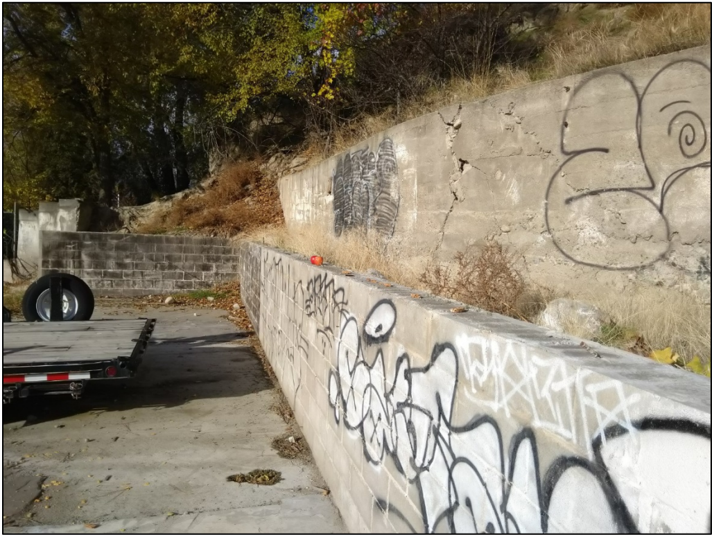
Figure 9: Existing Retaining Wall at rear of property
