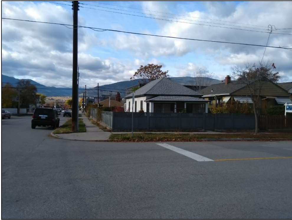
Figure 4: East View (from Van Horne Street)
