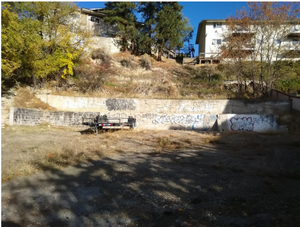
Figure 7: Rear Yard of Subject Property
