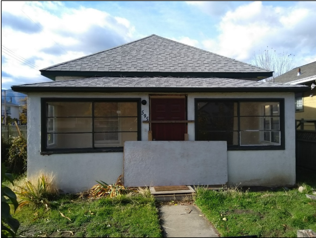
Figure 6: East View of the front of existing dwelling to be demolished
