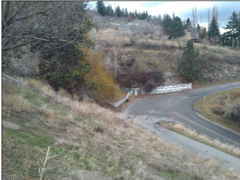
Figure 7: Slope at Intersection of Crescent Hill and Valleyview Road
