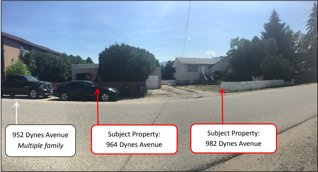
Figure 4 – Looking at front of 964 and 982 Dynes Avenue from Dynes Avenue
