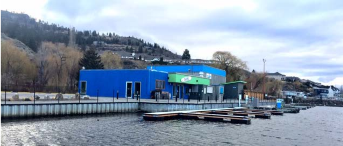
Figure 2 - North West side of the Building
