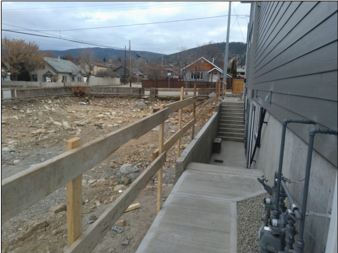
Figure 7: West View (showing proximity to new duplex to the south)
