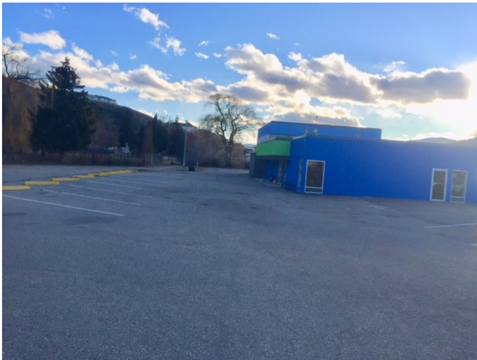
Figure 4 – Front and side of building, Storage and Parking Area
