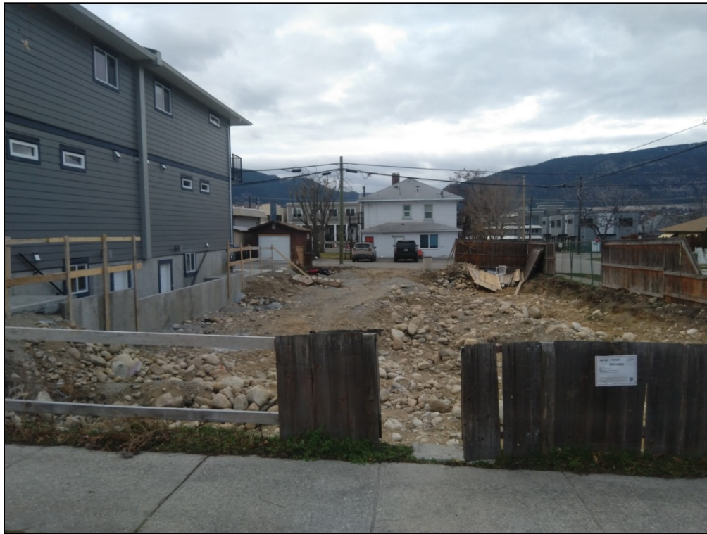
Figure 4: East View (from Van Horne Street)
