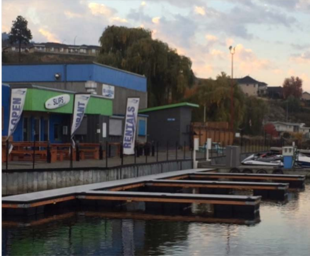
Figure 3 - back of the Building
