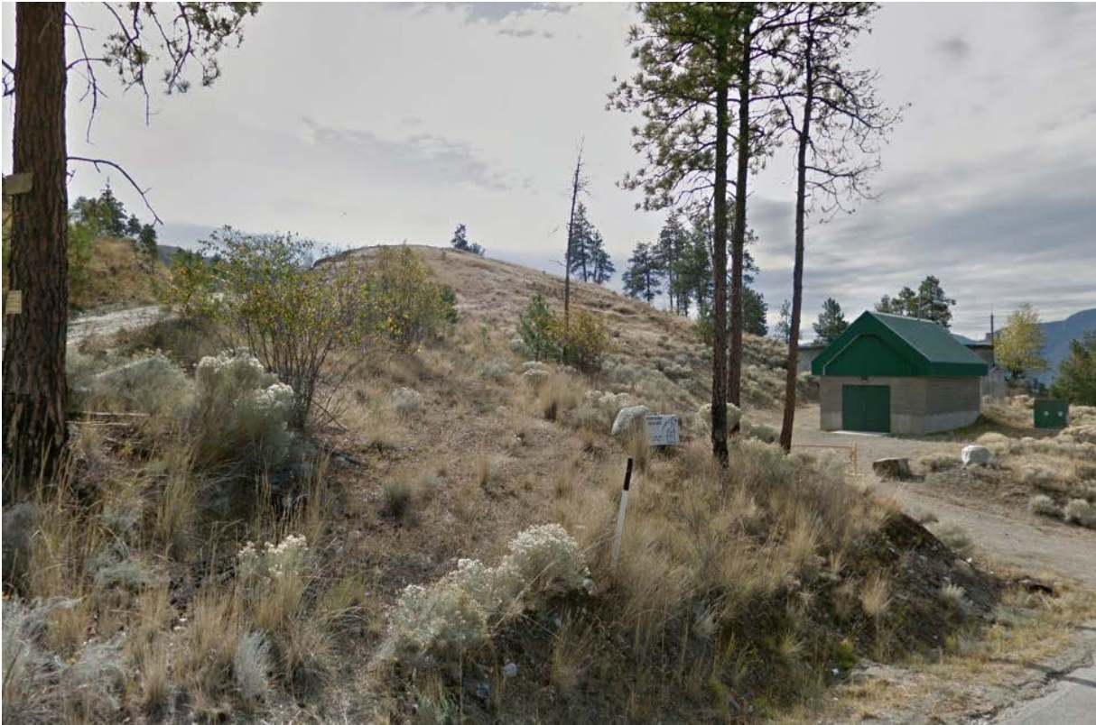
Figure 6: Looking west with water pump house in mid-ground
