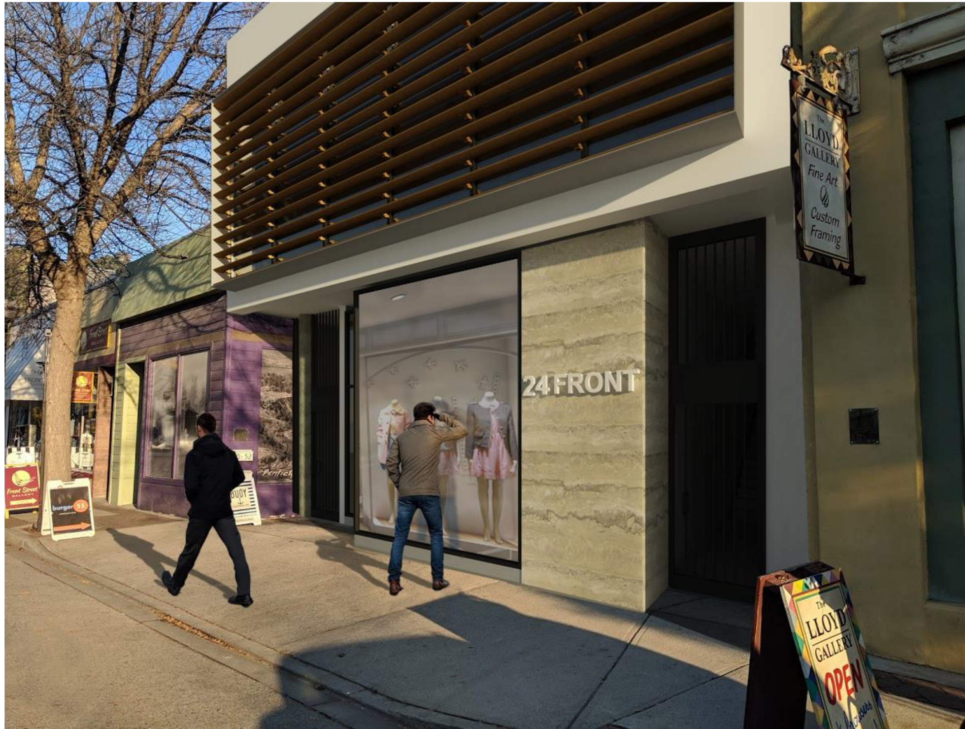
The building exterior materials were selected to be part of and enhance the fabric of Front Street. Large scale stone cladding adorns the retail / gallery storefront, while contrasting window frames and shimmering sunshade on the second floor sit boldly next to the finely crafted finish of the rest of the building.
