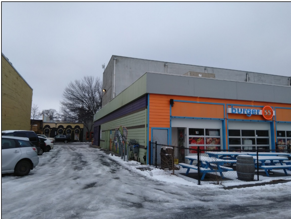
Figure 7: Lane View showing property to the North
