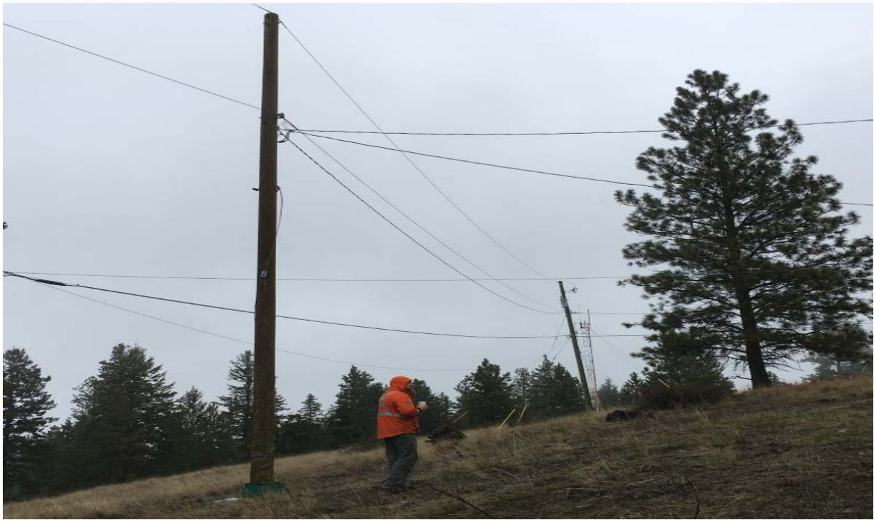
Figure 3: Photograph of the existing pole line
