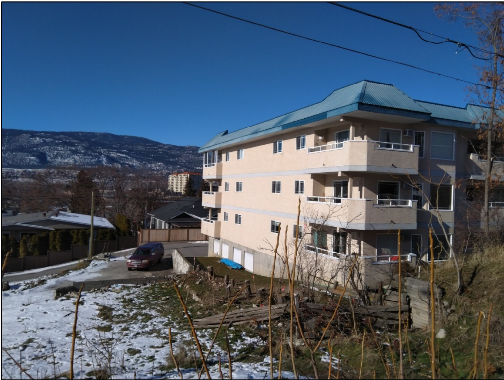
Figure 6: East View showing apartment building to the north
