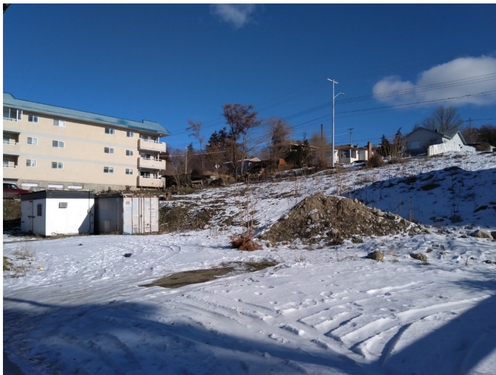
Figure 9: West View of Subject Property (from the lane)
