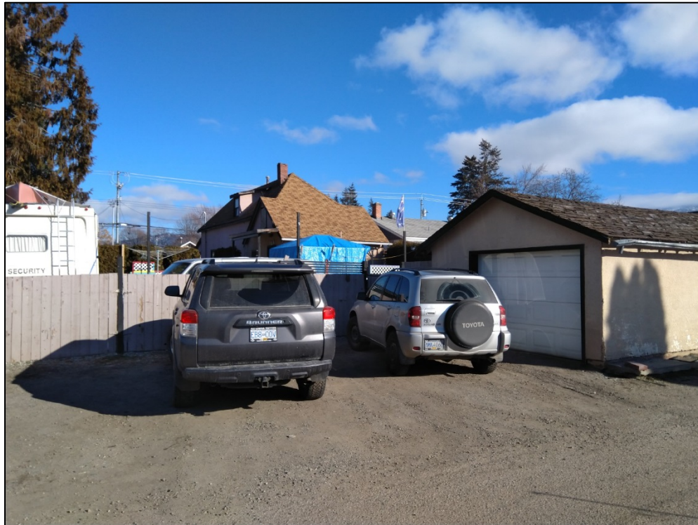
Figure 7: South View (from the lane)
