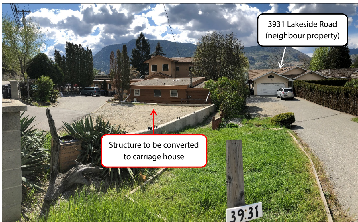
Figure 7 – Looking west toward subject property along northern property line
