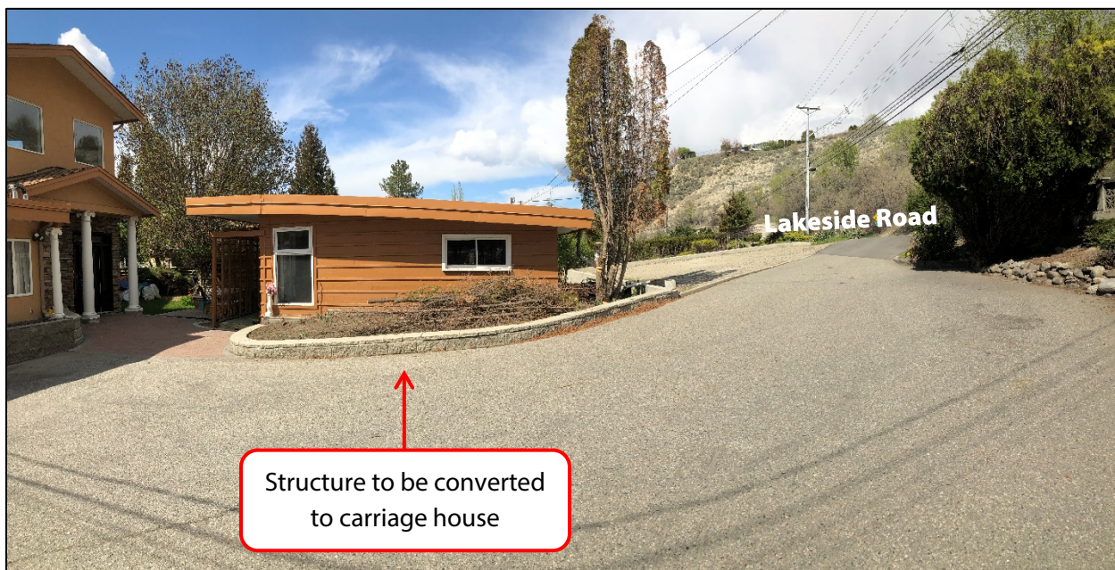
Figure 5 – Looking north at accessory building to be converted to carriage house
