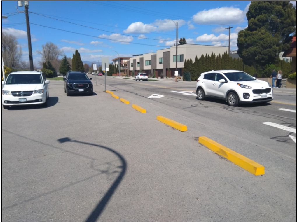
Figure 7: South View (looking along Power Street)
