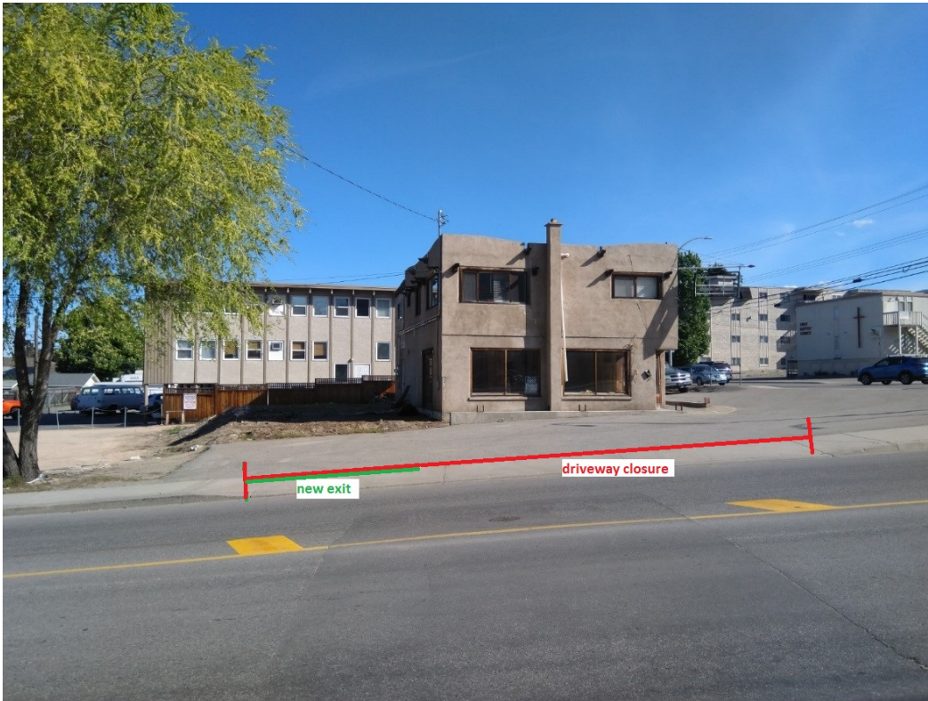
Figure 4: South view of subject property (from Carmi Avenue)
