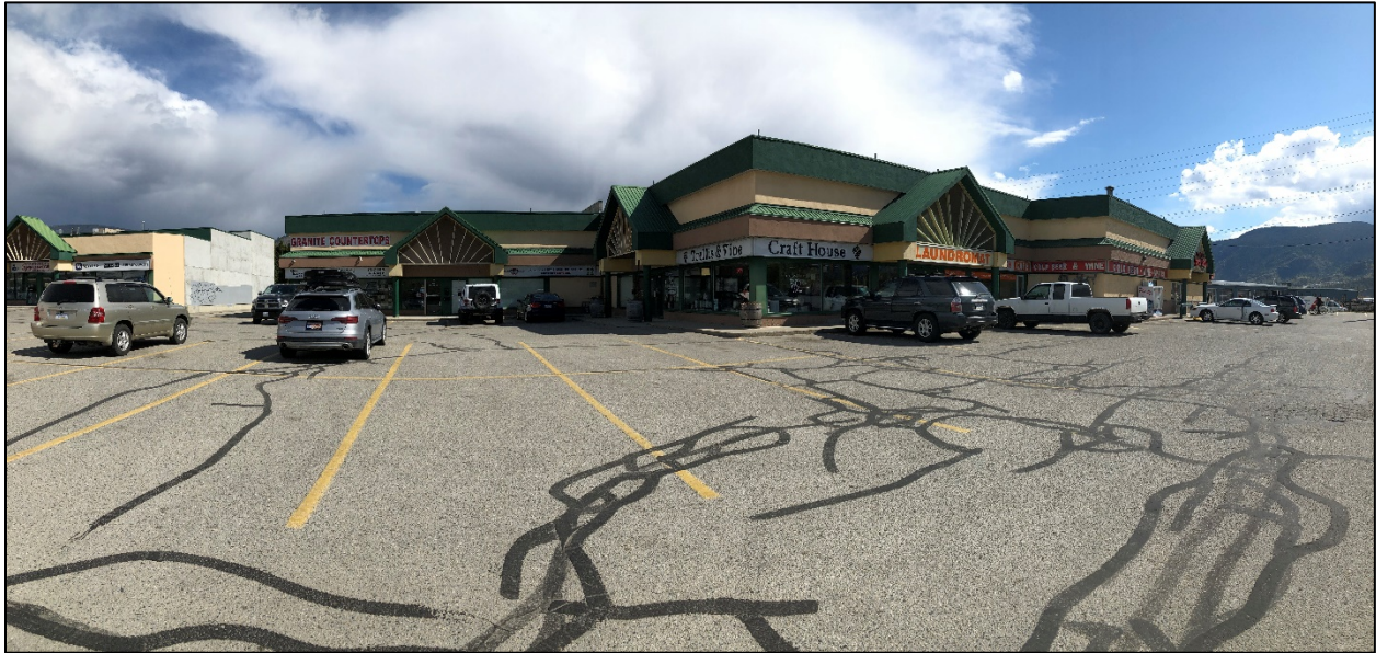
Figure 4 – Looking east towards strip mall building on subject property
