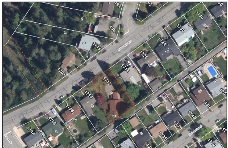
Figure 1 - Typically houses on Ridgedale Avenue are setback between 6-10m from the street
