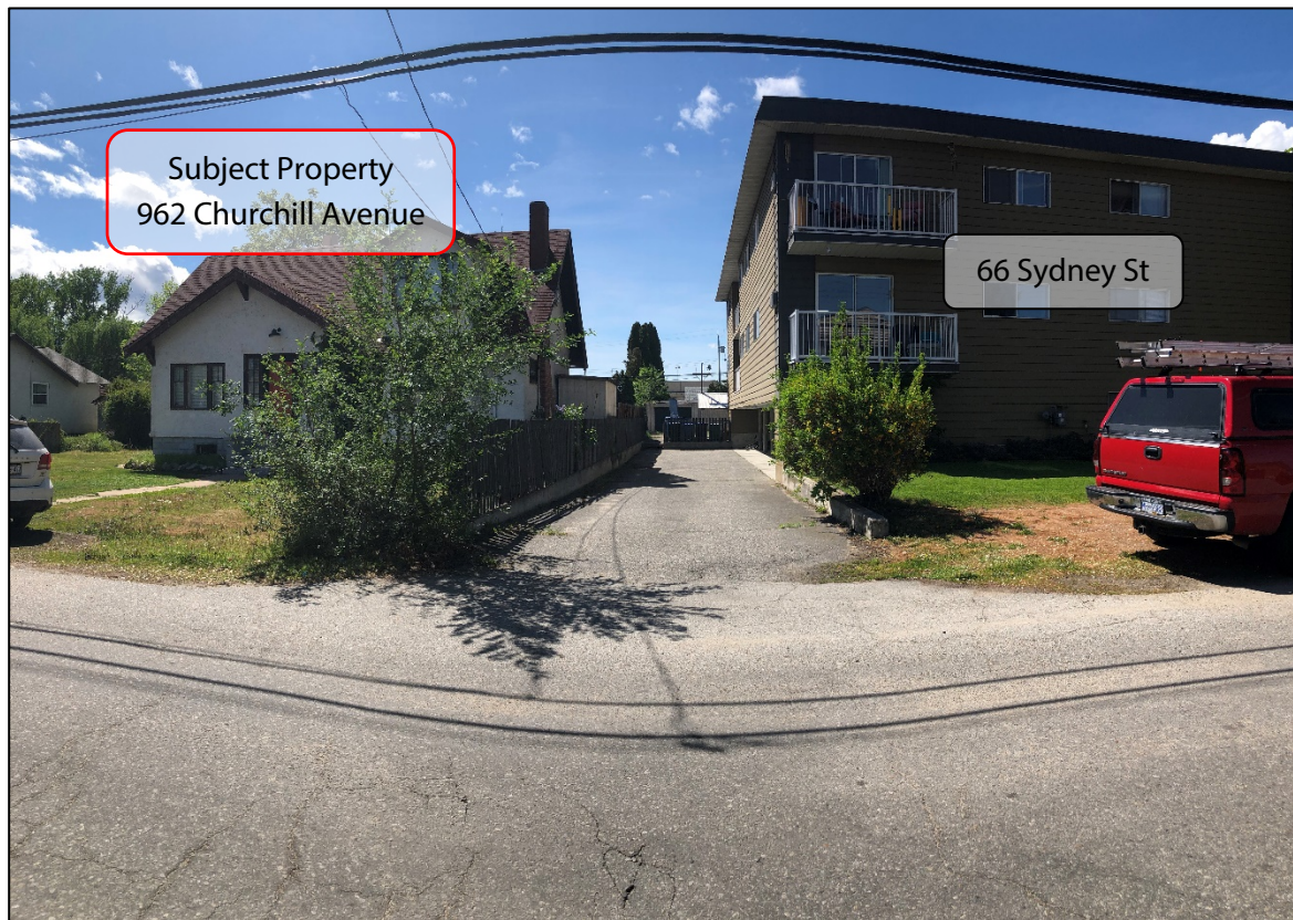
Figure 5 - Looking along western property line of subject property from Churchill Avenue
