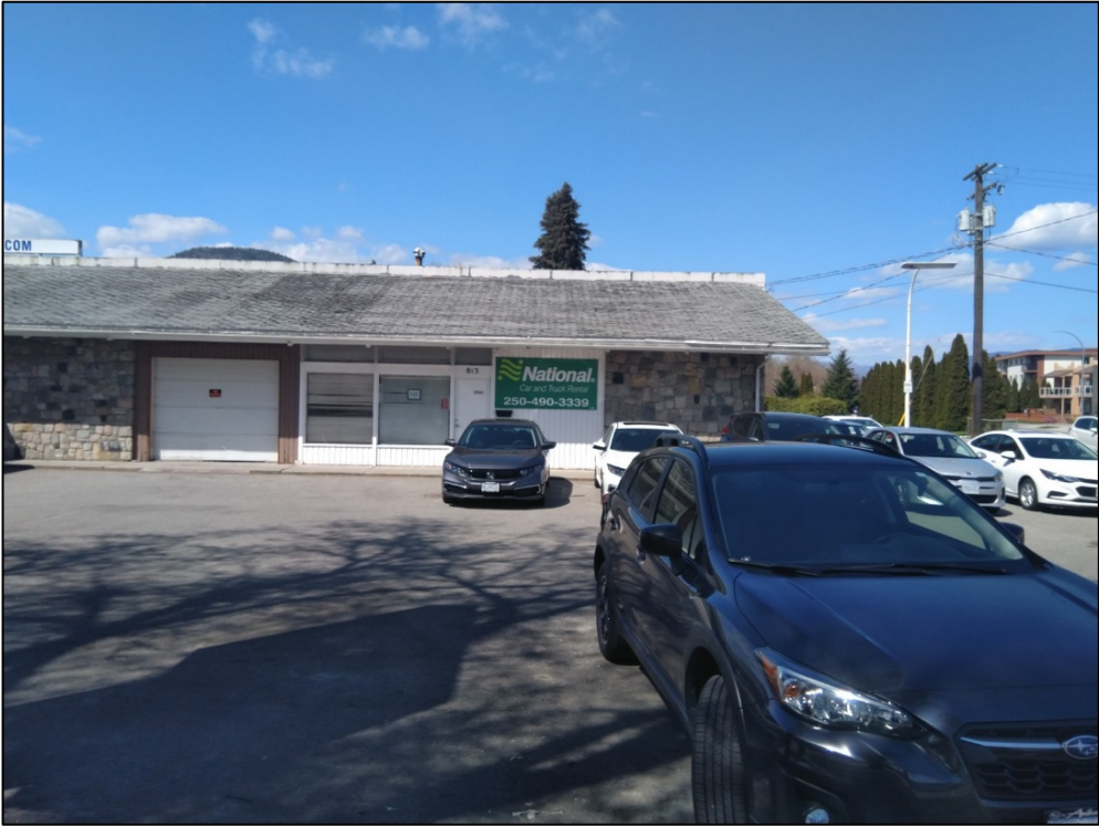
Figure 2 - South View (from Westminster Ave W)
