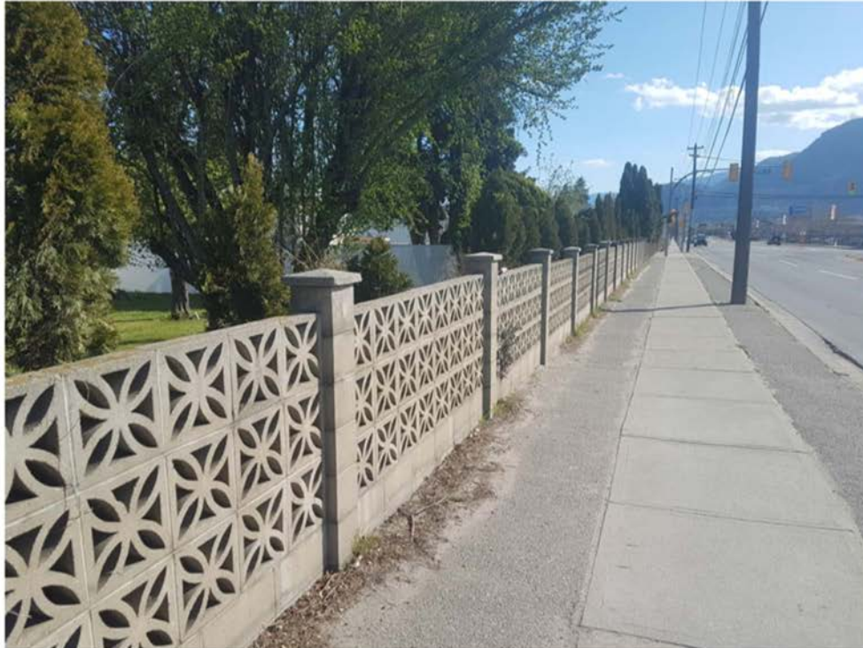
Image of Dauphin Park perimeter wall along Skaha Lake Road looking north showing Fairhaven 1.8 meter high steel fence next door.
