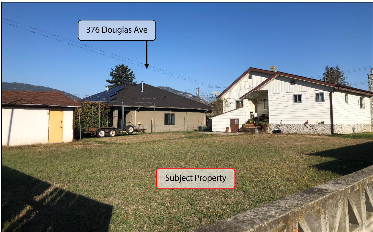
Looking into rear of subject property from laneway
