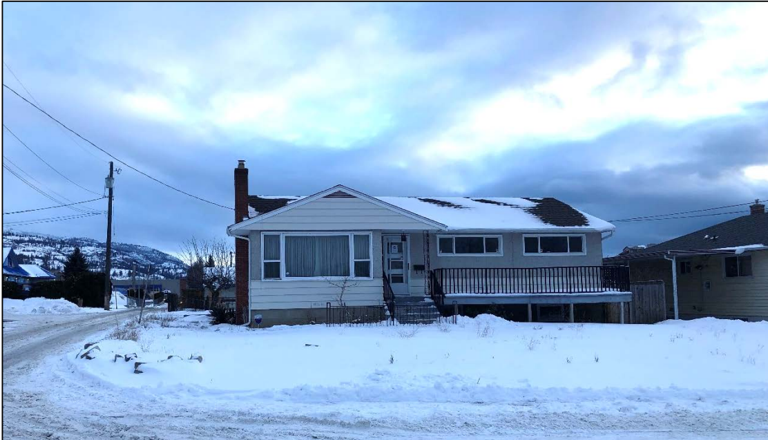
Looking south towards subject property from Okanagan Ave W
