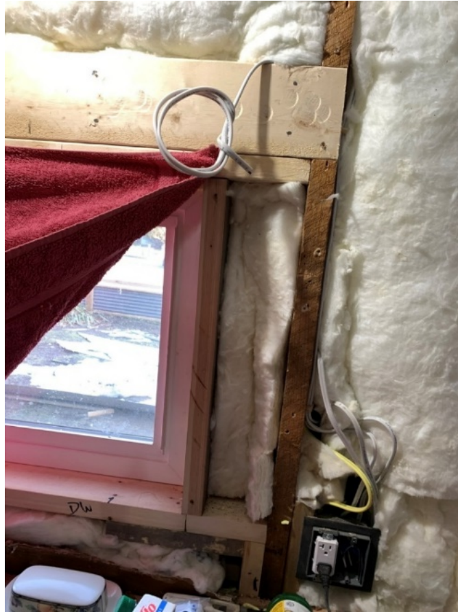
A photograph of the interior of an eastern front window of the single-family dwelling that required a king stud to be installed against a cripple stud.
