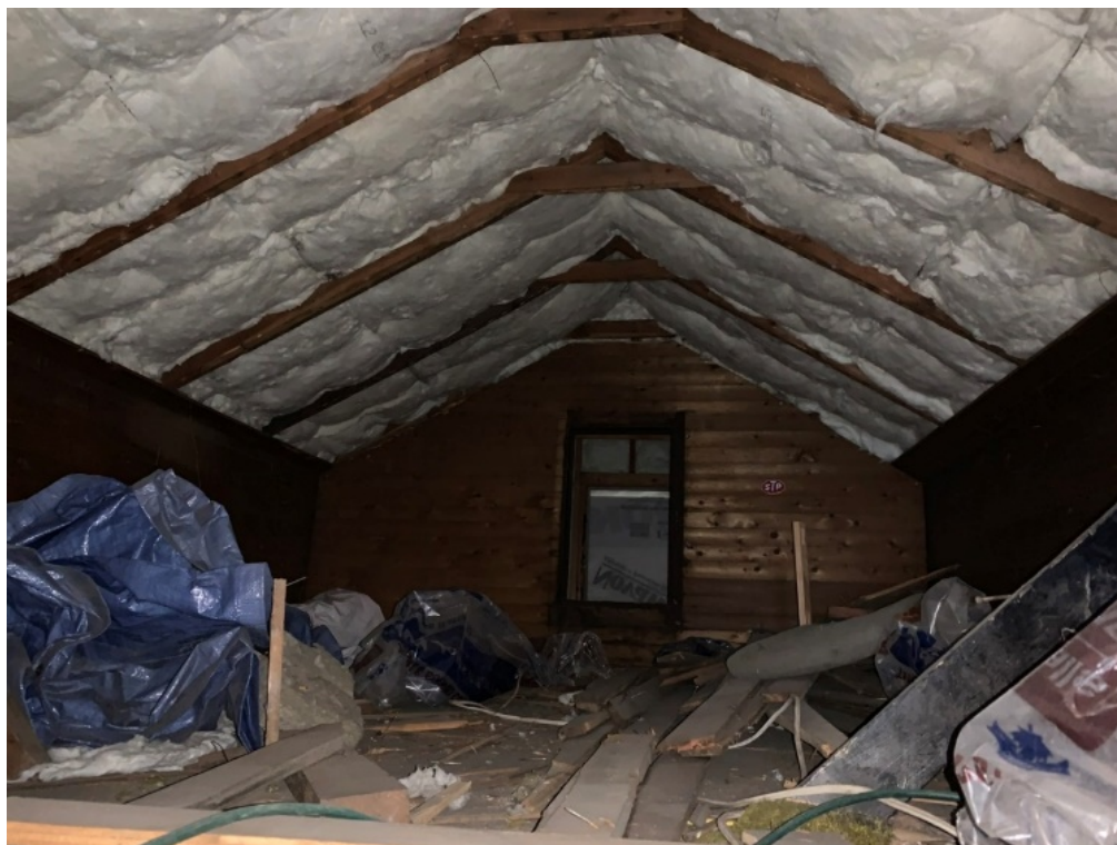
A photograph of the attic space of the single-family dwelling that appeared to be being finished for living space.
