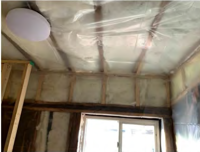
A third photograph of the interior of the bathroom group that shows the insulation of the exterior walls and in the ceiling of the low sloped roof. The insulation of the room was required meet the values given in the British Columbia Building Code and to be noted on the revised drawings.
