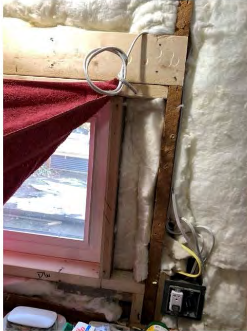
A photograph of the interior of an eastern front window of the single-family dwelling that required a king stud to be installed against a cripple stud.
