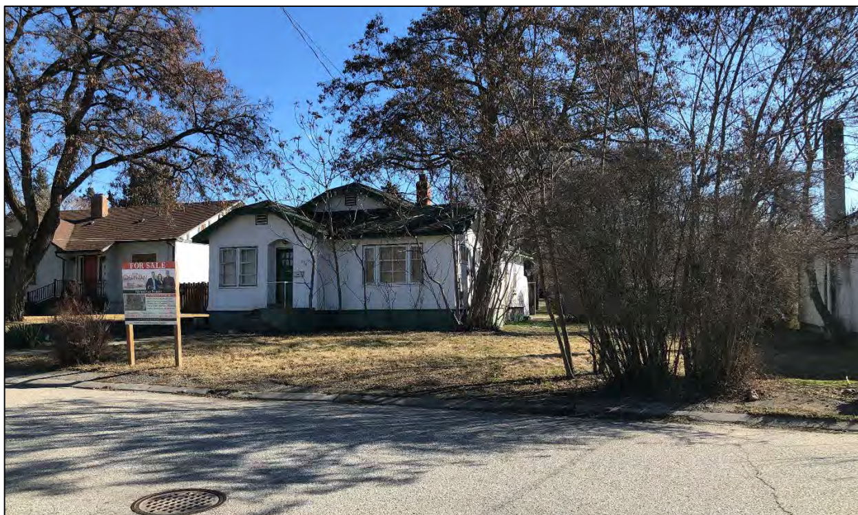
Looking towards subject property from Argyle St
