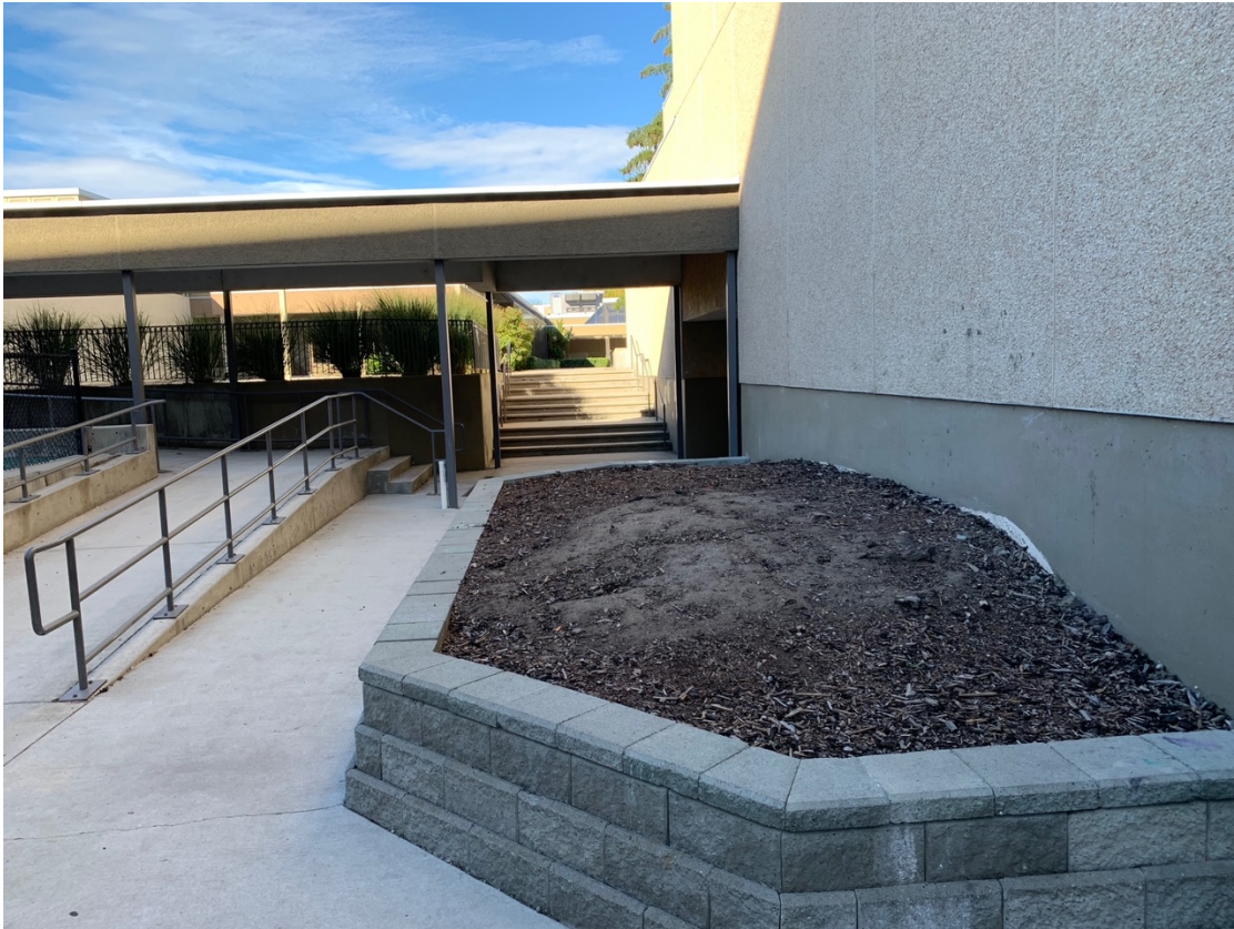
Image 3. Looking north beside the Community Centre; the PTCC is in the background
