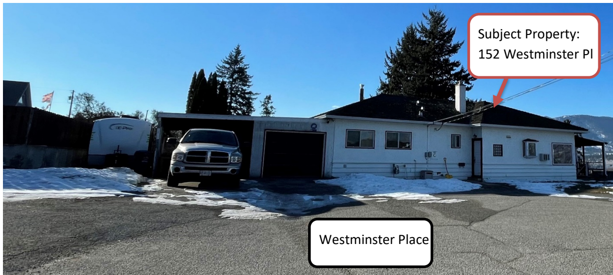
Looking south at the subject property from Westminster Place.
