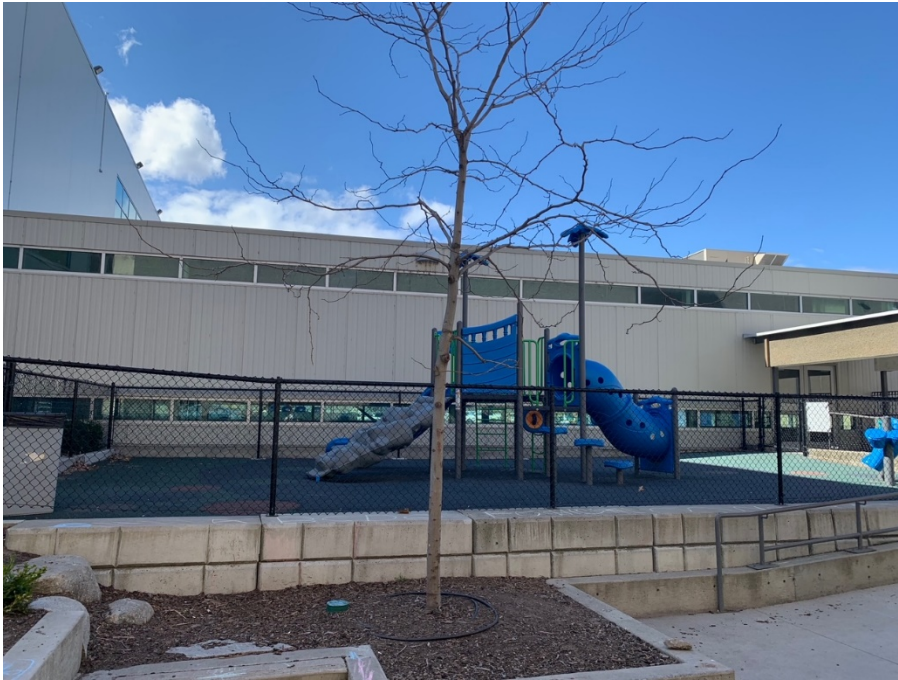
Image 1. Playground structure on the west side of the Community Centre
