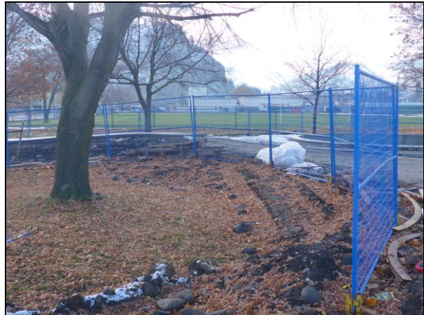
Above: Examples of suitable fencing made from chain link, 4 to 6 feet high, anchored.
