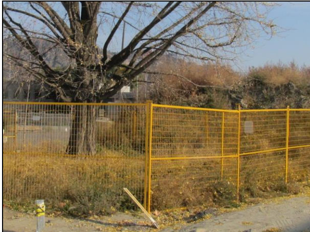
Above: Examples of suitable fencing made from chain link, 4 to 6 feet high, anchored.
