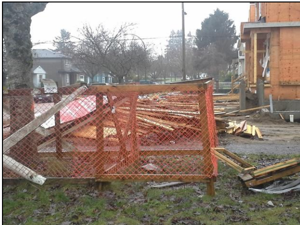
Above left: Example of suitable fencing made from 2x4 wood and snow-fencing.
