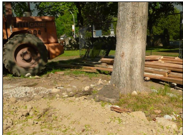
Above left: Most tree roots important for uptake of water and food are found in the top 15 to 30 cm of soil and extend to an area just past the dripline from the tree canopy.
