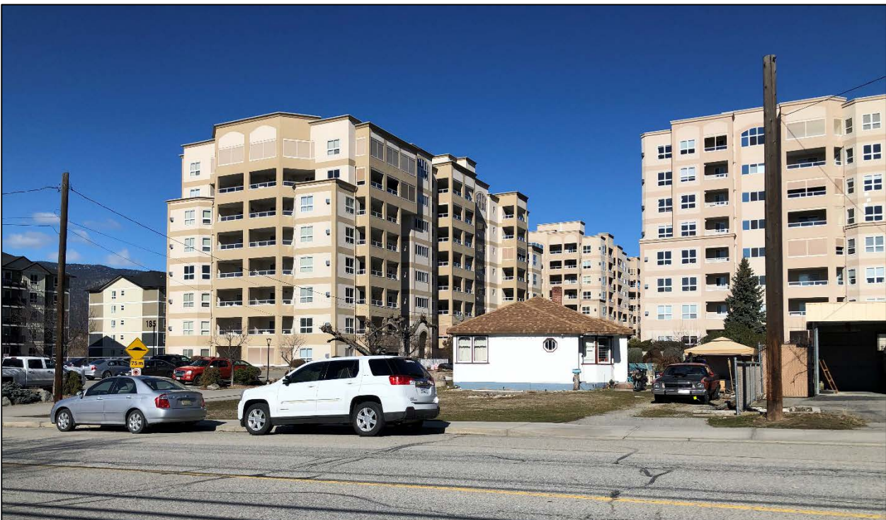
Looking north at subject property from Kinney Avenue
