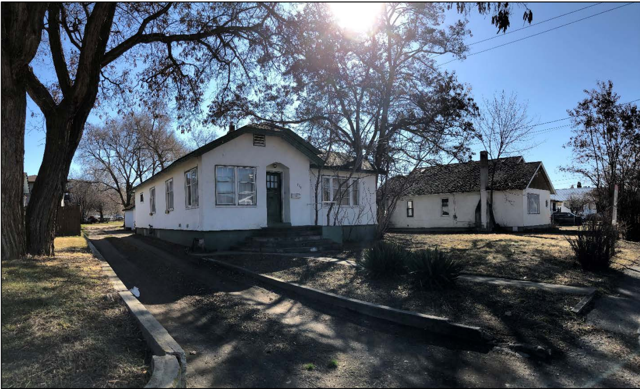
Looking towards subject property from Argyle St
