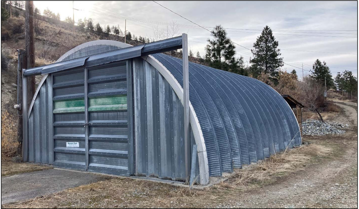
Existing accessory structure (Quonset hut) proposed to be converted to carriage house
