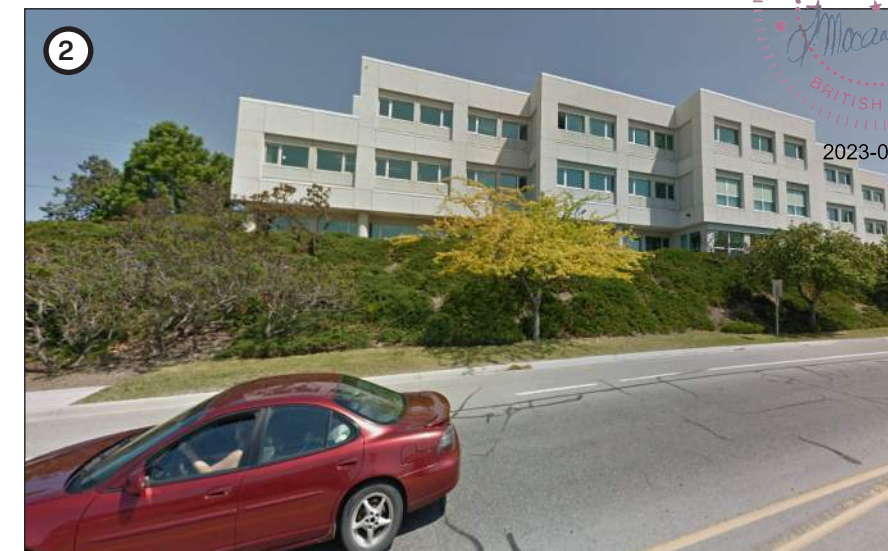
View of the 740 Carmi Ave, fronting onto Government St.
